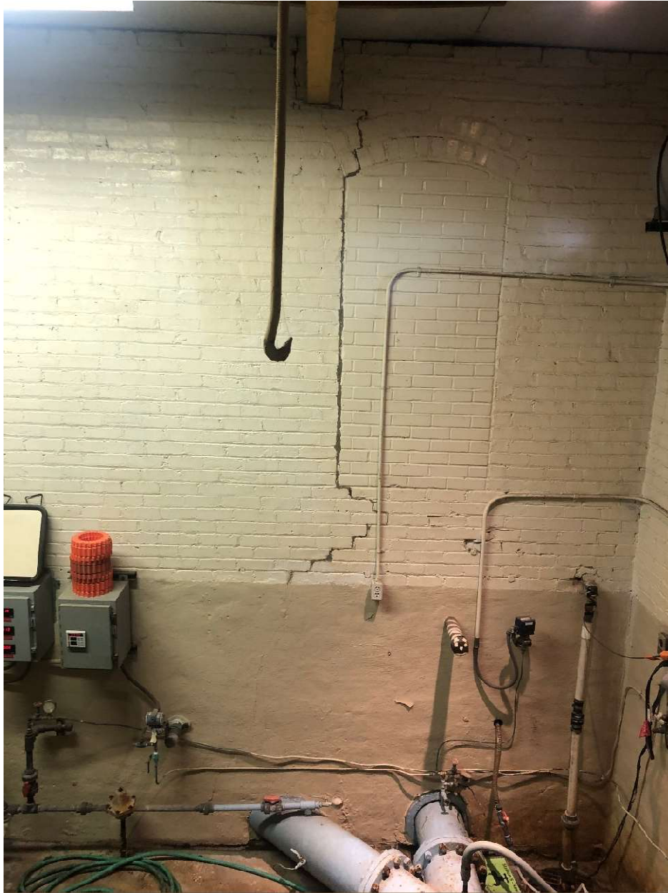
Proposed Structural Steel Vertical Load Support Column – West Column Proposed Location – See Structural Steel Specs – Place W16 x 26 105" from Existing Floating Beam to New Proposed Concrete Pier Placed 60" Above Basement Floor.
