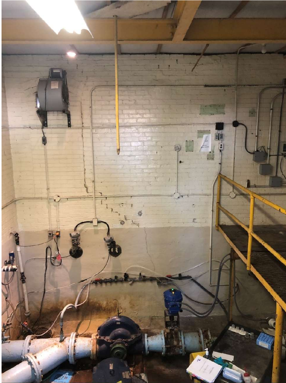
Interior North Elevation – Facing North
