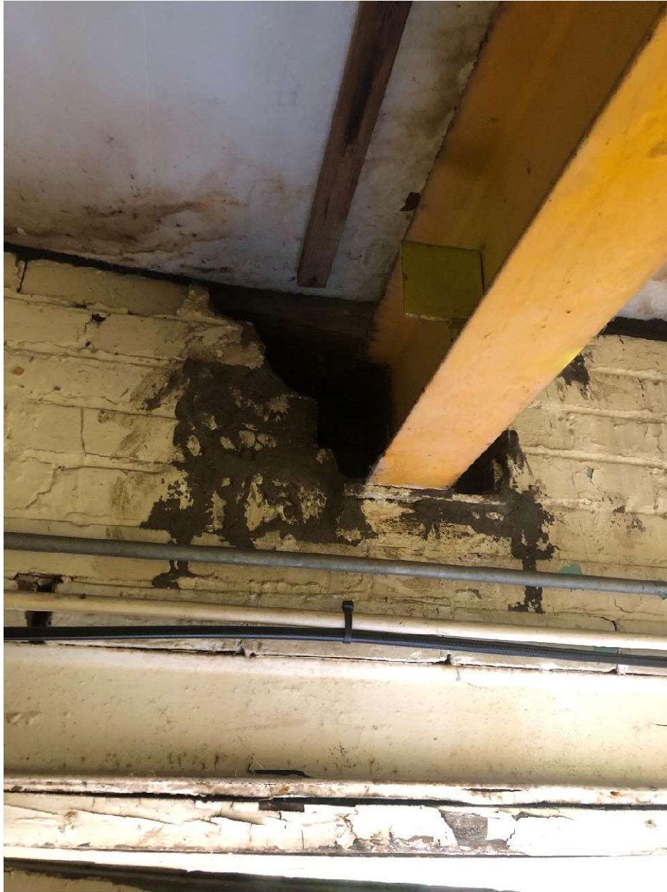
Interior South Elevation – Facing South – Detail View
