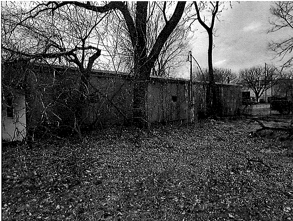
View of the right side of the building (EA-4)
