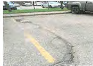
Crackfill needed
