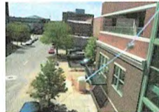
Hole and crack in crosswalk
