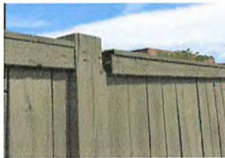
Fix dumpster wall
