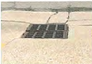
Check drain for damage
