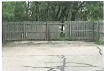
Clean and repair fence
