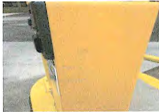
Clean and touch up paint
