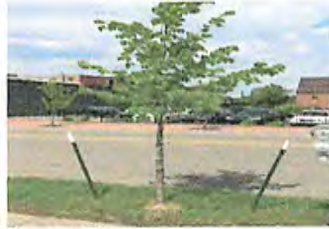
Remove tree stakes
