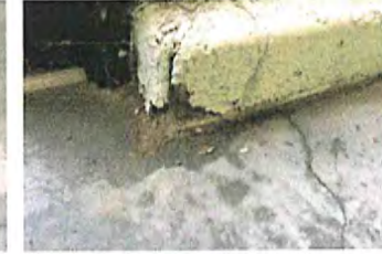
East stair door
