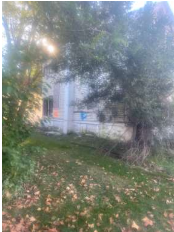
View of the left side of the house (EA-2)
