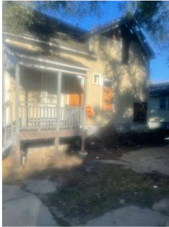
View of the rear of the house (EA-3)
