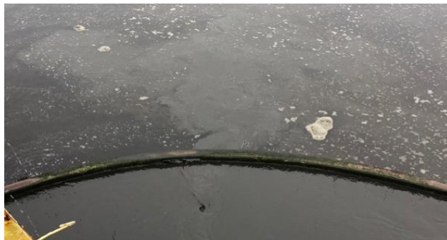
MLSS Flowing Out of Scum Port
