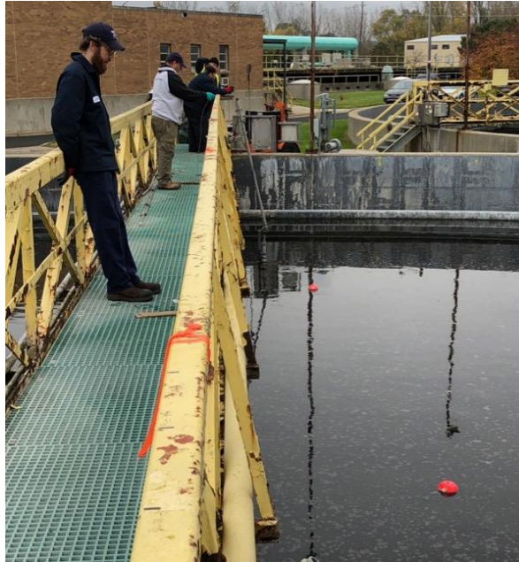
Monitoring Drogues in a Clarifier
