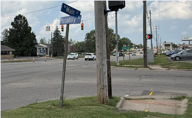
Intersection of West Main Street and Piccadilly Road, showing wide auto-oriented design and frequent driveways that contribute to turning conflicts and lack of connected and accessible pedestrian infrastructure.
