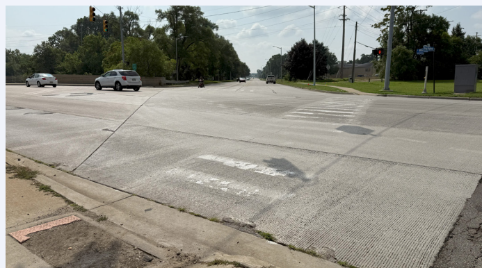
Faded crosswalk and deteriorated curb ramp at East Michigan Avenue and Amvets Memorial Parkway, showing accessibility and visibility challenges.
