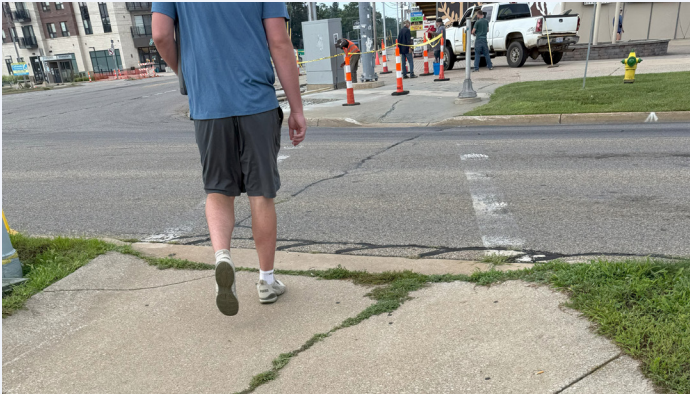
Damaged and uneven pedestrian island, missing tactile warnings, and worn crosswalk across Howard Street at the intersection with West Michigan Avenue.
