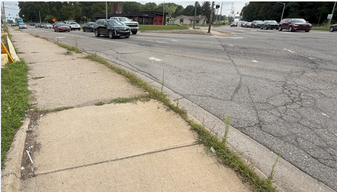
Long crossing distance, missing curb ramps, and deteriorated sidewalks and crosswalk striping.
