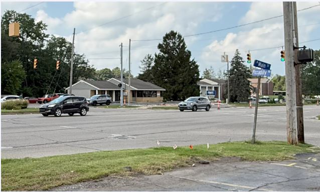
Wide view of West Main Street and Piccadilly Road, highlighting commercial driveways, wide crossing distances, and lack of pedestrian-scale infrastructure.
