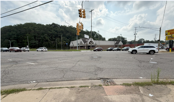
Wide and cracked pavement crossing at the south leg of Riverview Drive and Gull Road intersection in Kalamazoo. Also, faded crosswalk and non-directional curb ramp, very wide radius.
