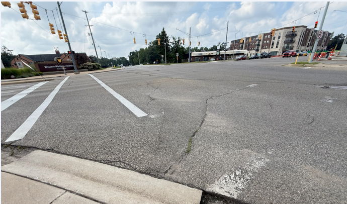
Uneven, non-ADA compliant curb ramp and deteriorated pavement at the north crosswalk of Howard Street at the intersection with West Michigan Avenue.
