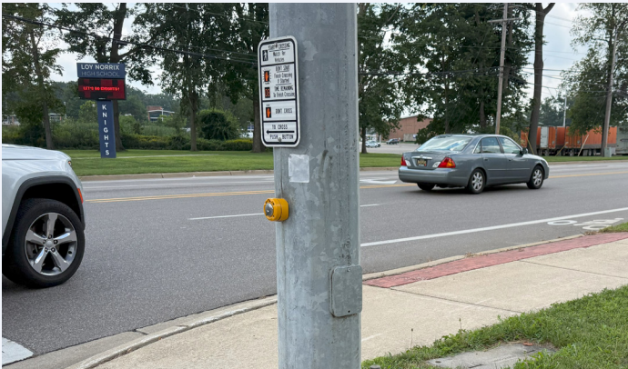
Pedestrian push button at Kilgore Road and Lovers Lane, showing obstructions and limited accessibility at the curb ramp.
