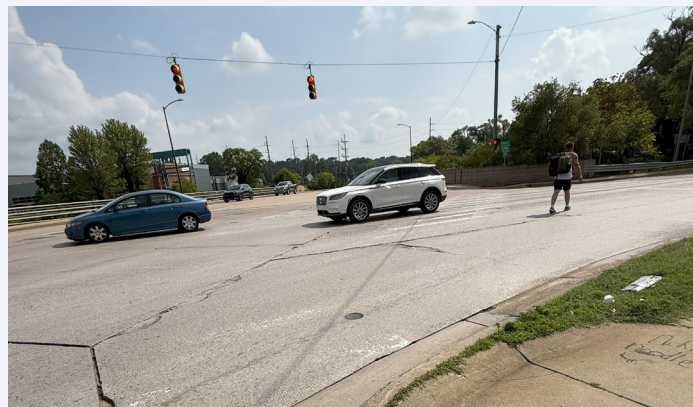
Pedestrian crossing East Michigan Avenue at Amvets Memorial Parkway, illustrating long crossing distances and lack of ADA-compliant curb ramps and faded crosswalk striping.
