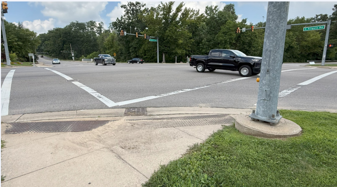
Curb ramp and crosswalk at Kilgore Road and Lovers Lane, illustrating deteriorated conditions and accessibility barriers for pedestrians.
