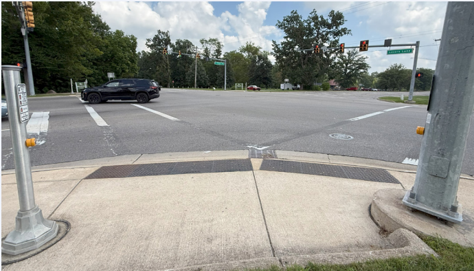
Wide view of the Kilgore Road and Lovers Lane intersection, illustrating long pedestrian crossing distances and a wide, auto-oriented layout.
