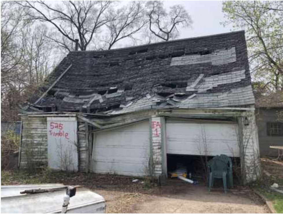
View of the garage located at 525 Trimble Avenue (EA-1)
