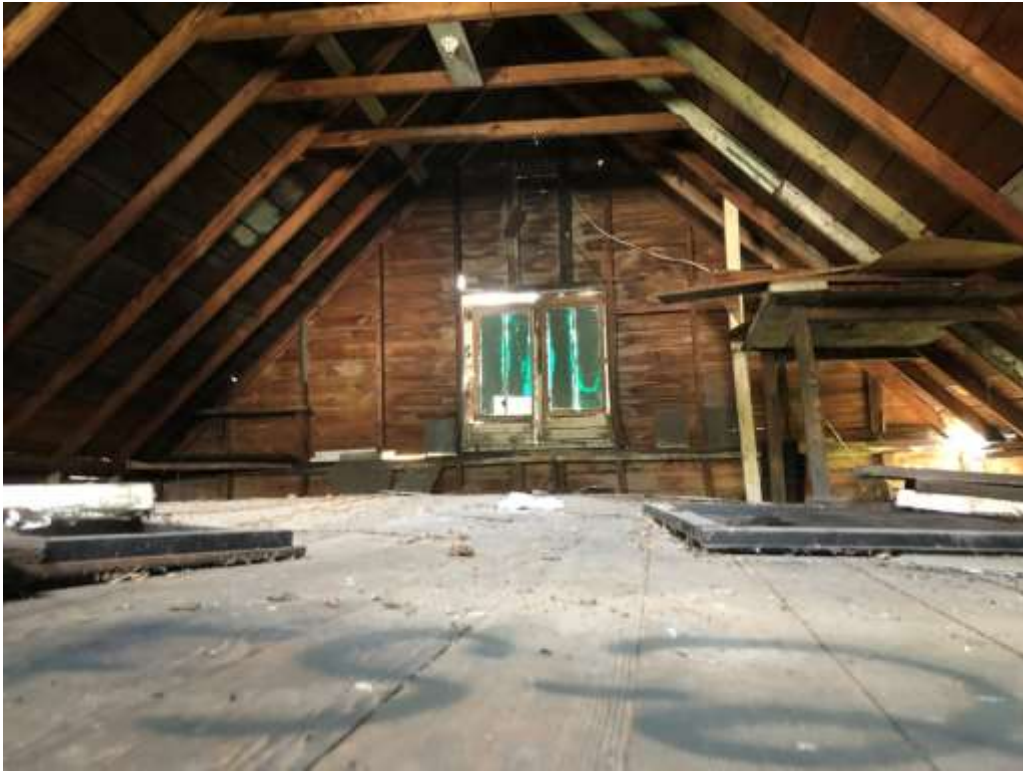
View of the garage attic (FS-2)
