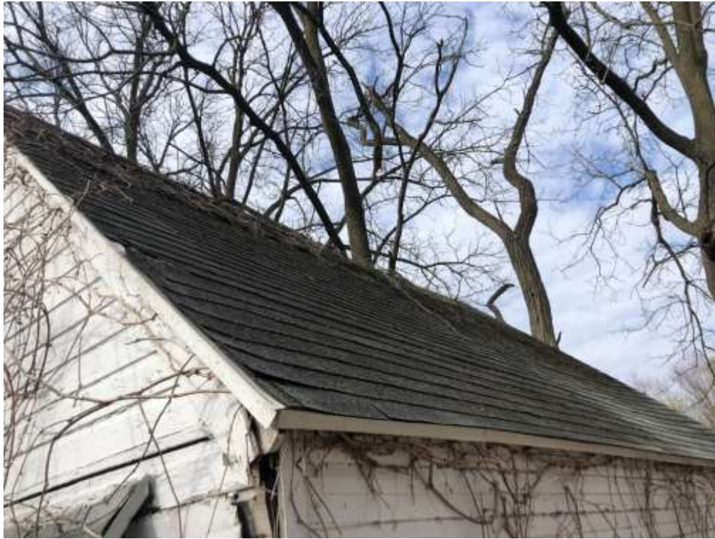
View of the roof (EA-5)
