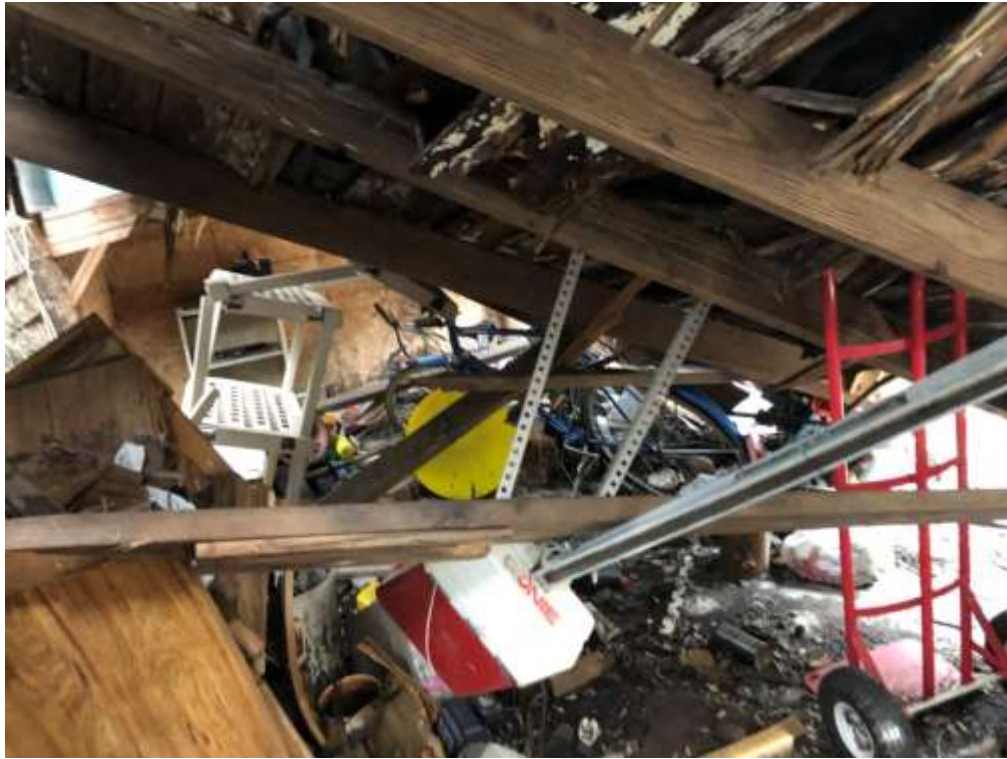
View of the garage interior (FS-1)
