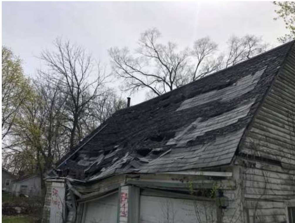
View of the roof (EA-5)
