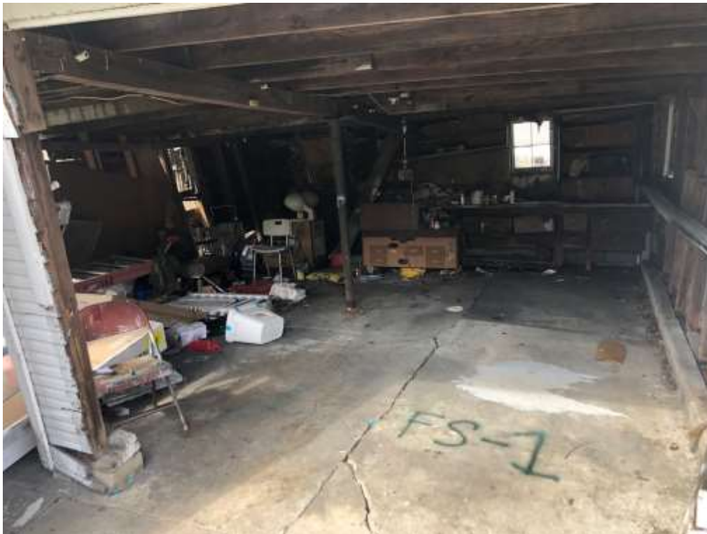
View of the garage interior (FS-1)
