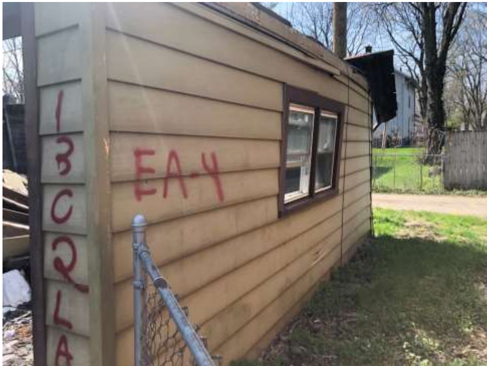
View of the right side of the garage (EA-4)
