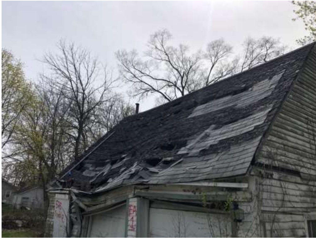
View of the roof (EA-5)
