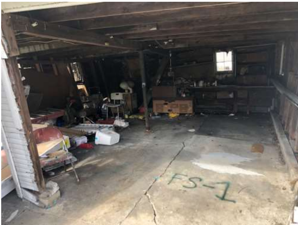
View of the garage interior (FS-1)
