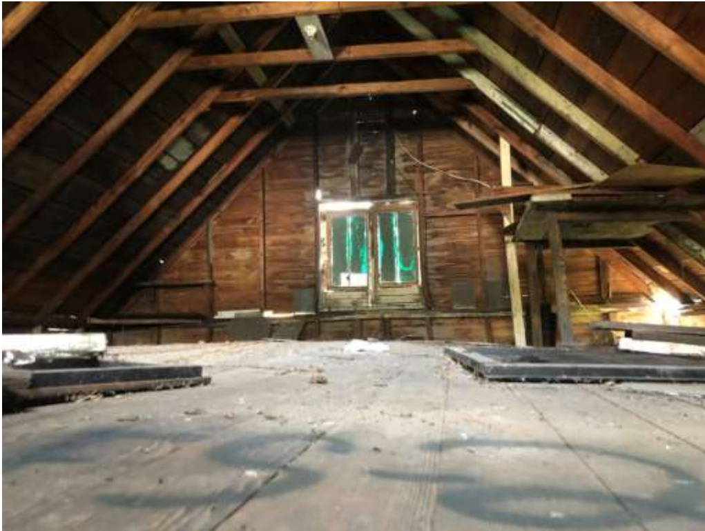
View of the garage attic (FS-2)
