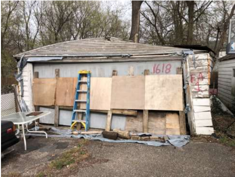
View of the garage located at 1618 N. Park Street (EA-1) and roof (EA-5)
