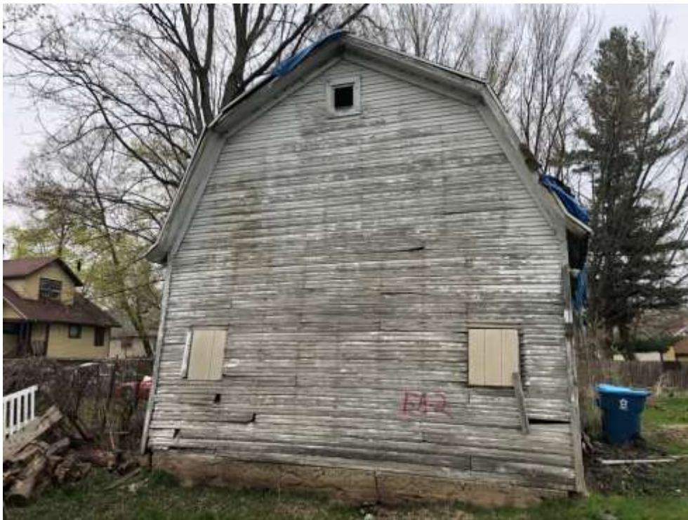
View of the left side of the garage (EA-2)
