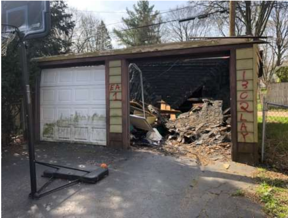
View of the garage located at 1302 Lay Boulevard (EA-1)
