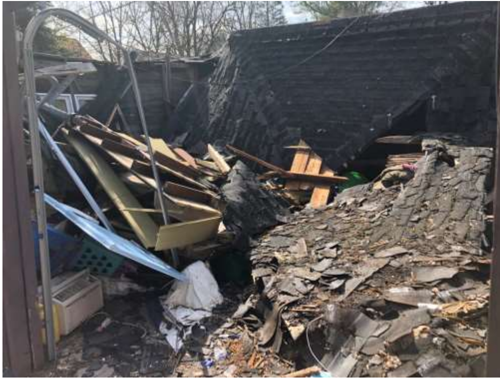
View of the roof (EA-5) and garage interior (FS-1)
