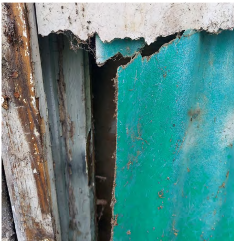
Window With Caulk and Glaze, Front of Structure (Close-Up)
