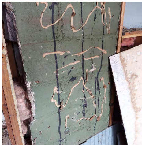
Black Wall Mastic, Room 2
