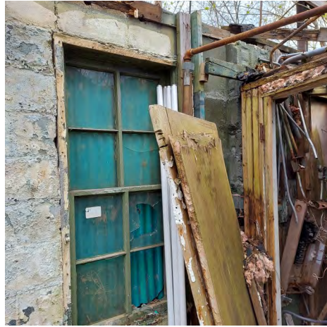
Window With Caulk and Glaze and Fluorescent Light Bulbs, Exterior
