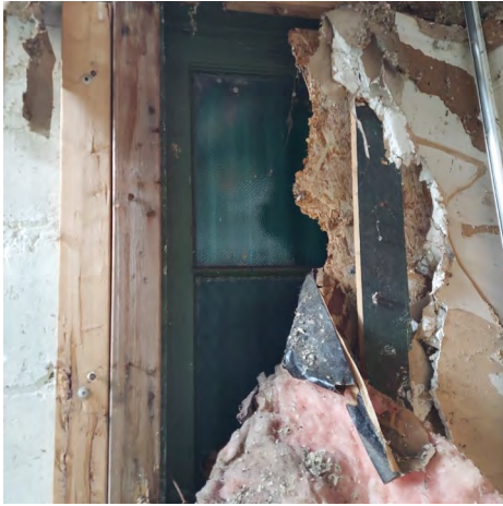
Window With Caulk and Glaze, Room 2
