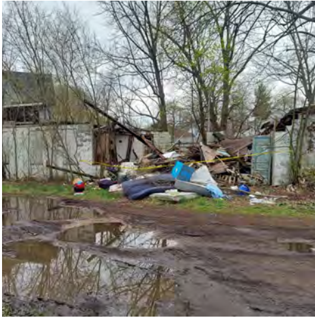
Front of Structure (From Driveway Approach)
