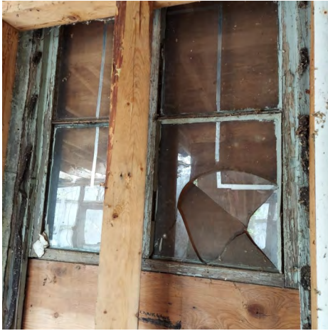
Windows With Caulk and Glaze, Room 4
