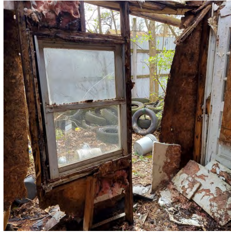
Window With Caulk and Glaze, Room 4
