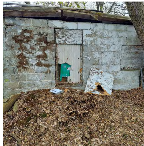
Window With Caulk and Glaze, Front of Structure (Step-Back)
