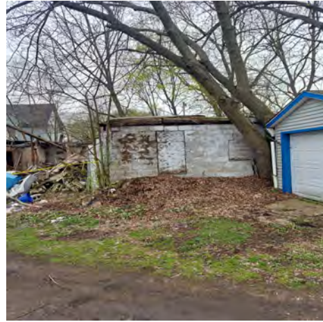
Front of Structure (Near Adjacent Property Owner's Garage)
