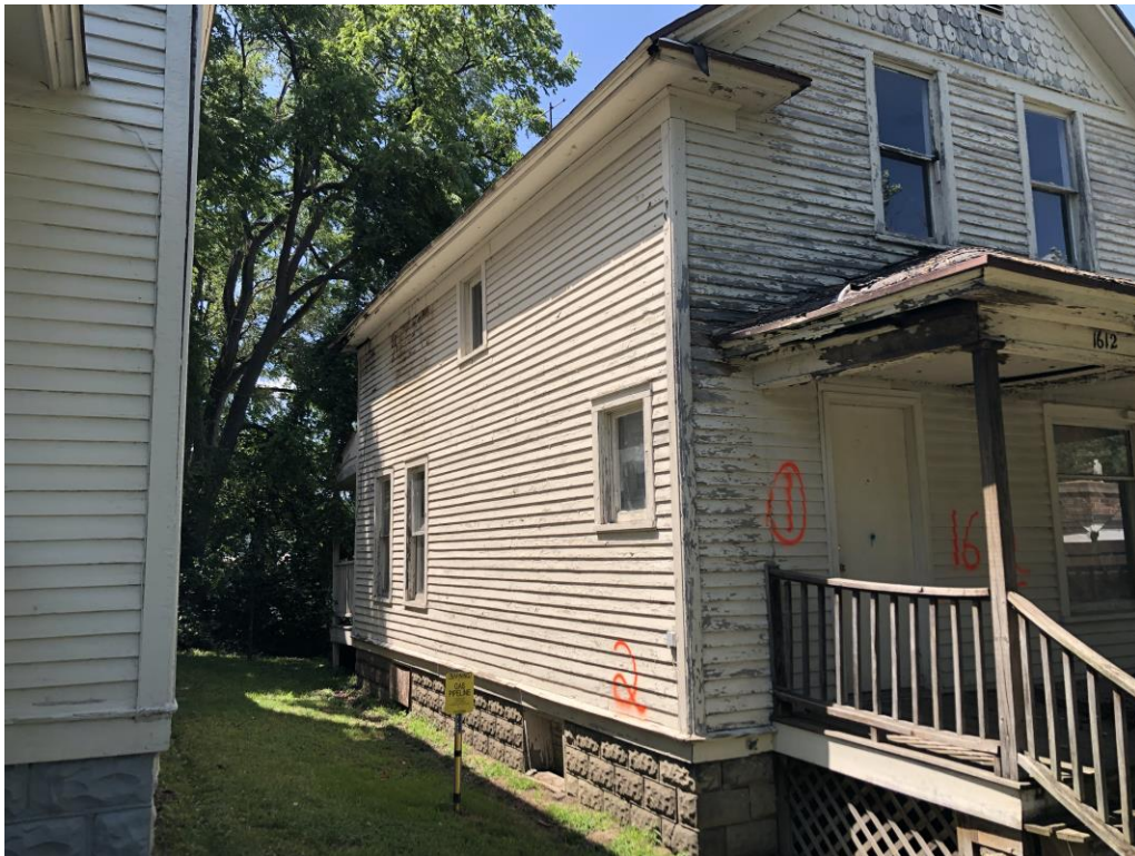
View of the left side of the house (EA-2)
