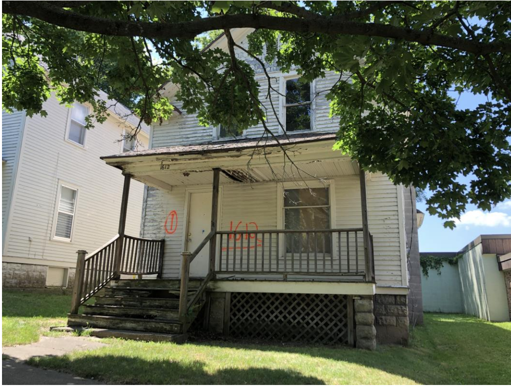
Street view of the house located at 1612 S Park Street (EA-1)
