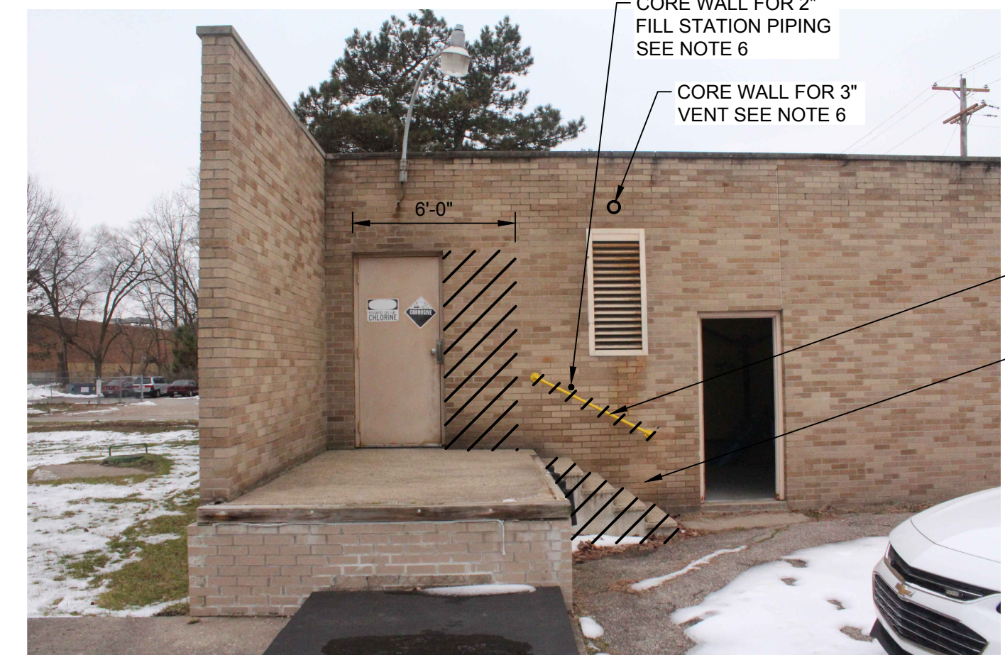
PHOTO 3-3 - PHOSPHATE FILL STATION
