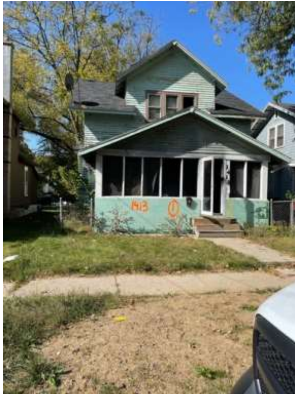
Street view of the house located at 1413 N Edwards (EA-1)/ (EA-5)
