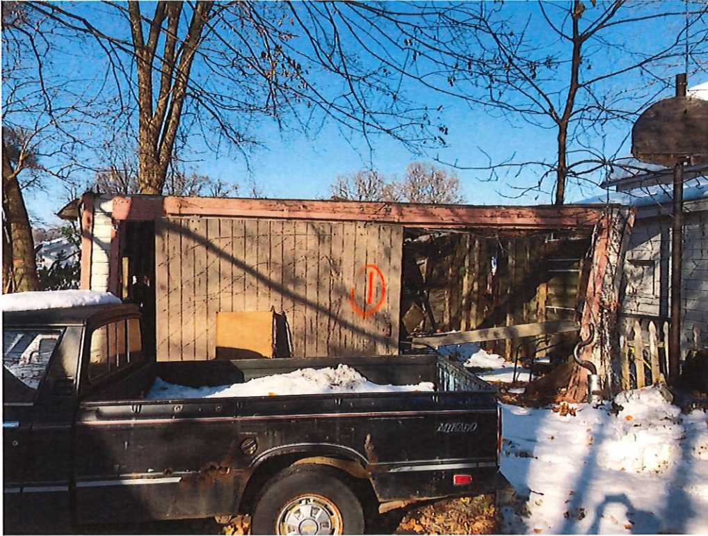
Street view of the garage (EA-1)
