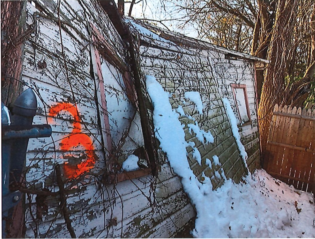
View of the rear of the garage (EA-3)
