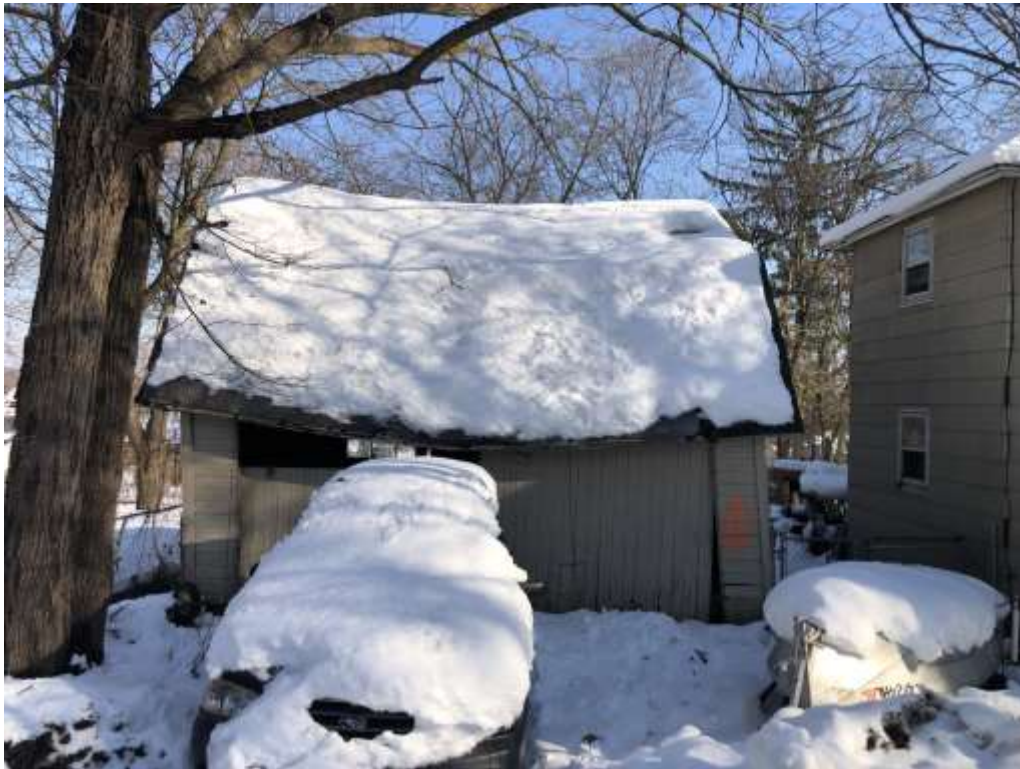
Street view of the garage (EA-1)
