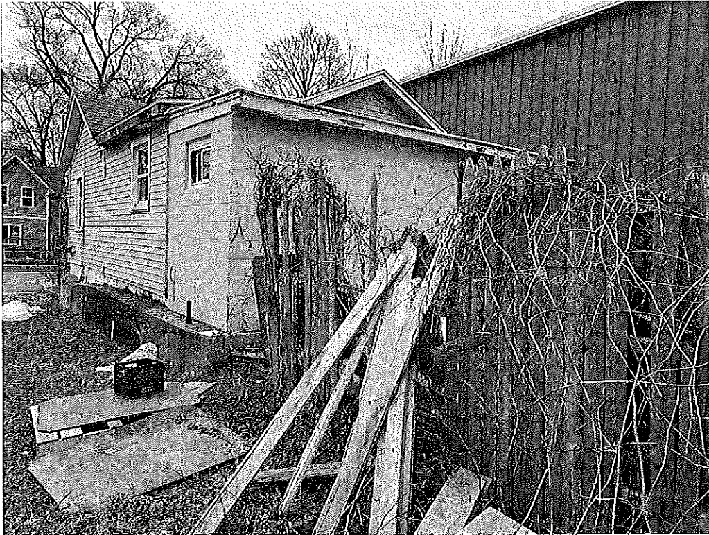
View of the rear of the house (EA-3)
