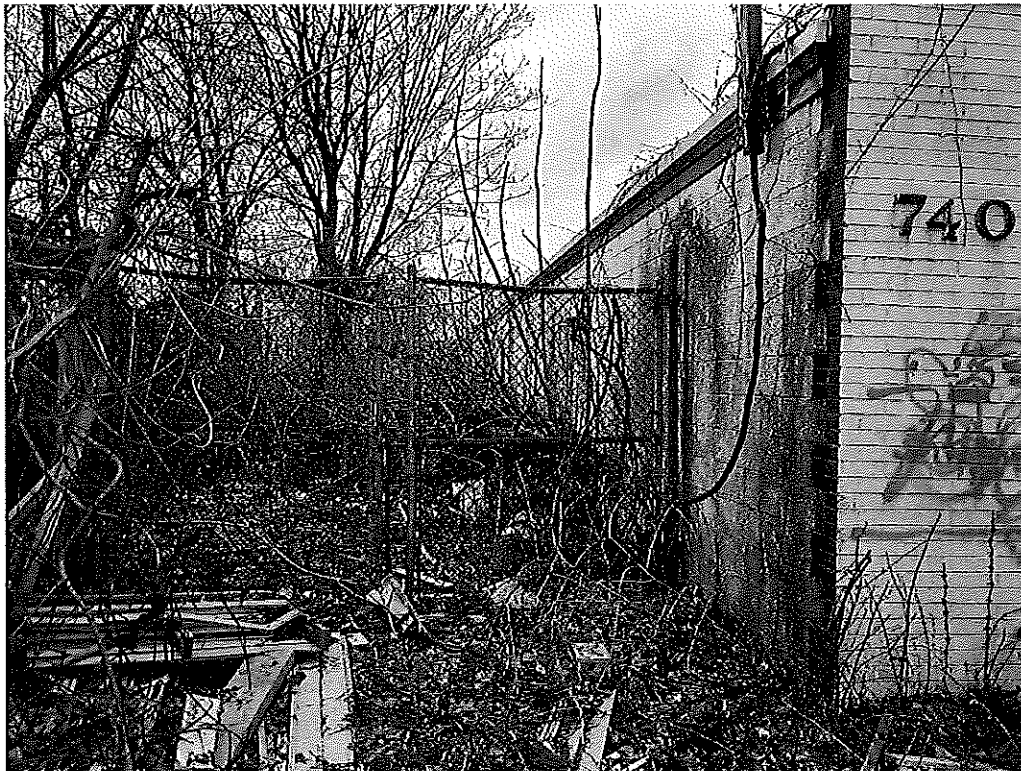
View of the left side of the building (EA-2)
