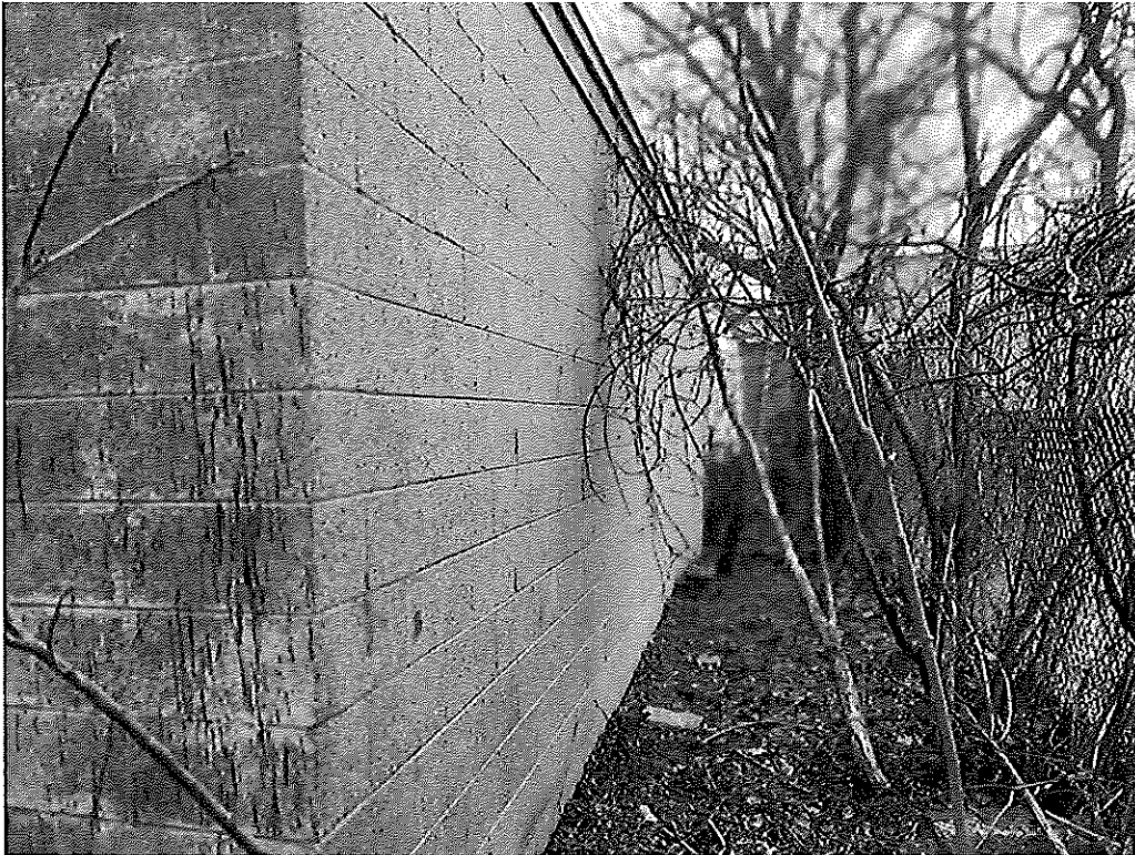
View of the rear of the building (EA-3)
