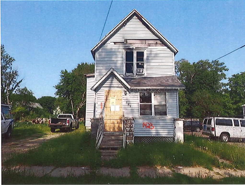
Street view of the house located at 1423 N Edwards (EA-1)/(EA-5)
