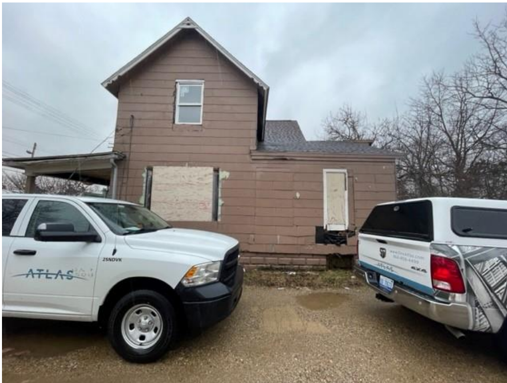
View of the right side of the house (EA-4)
