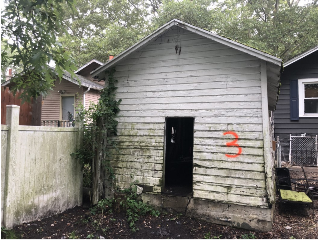
View of the east side of the garage exterior (EA-3)
