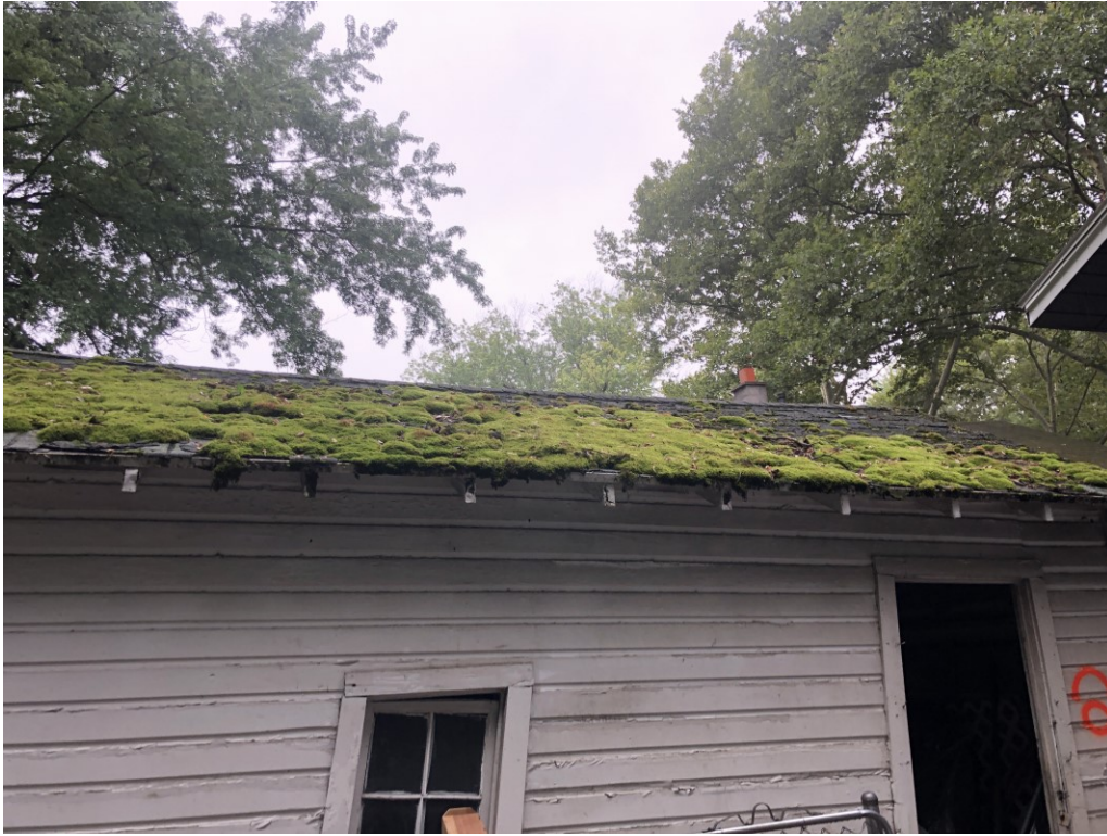
View of the garage roof (EA-5)
