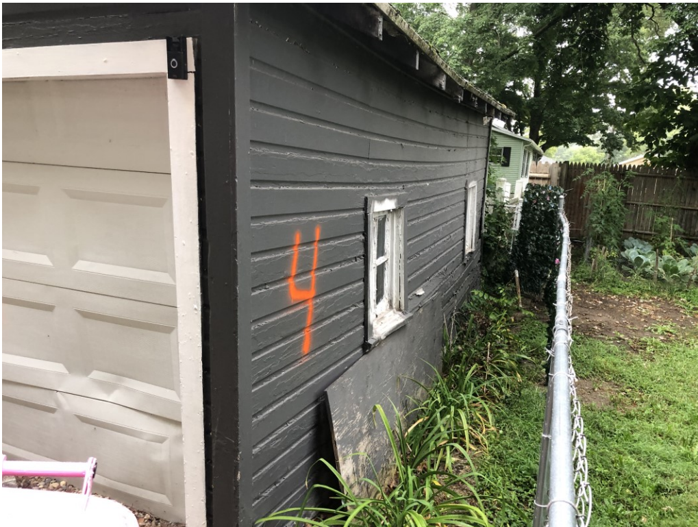
View of the south side of the garage exterior (EA-4)
