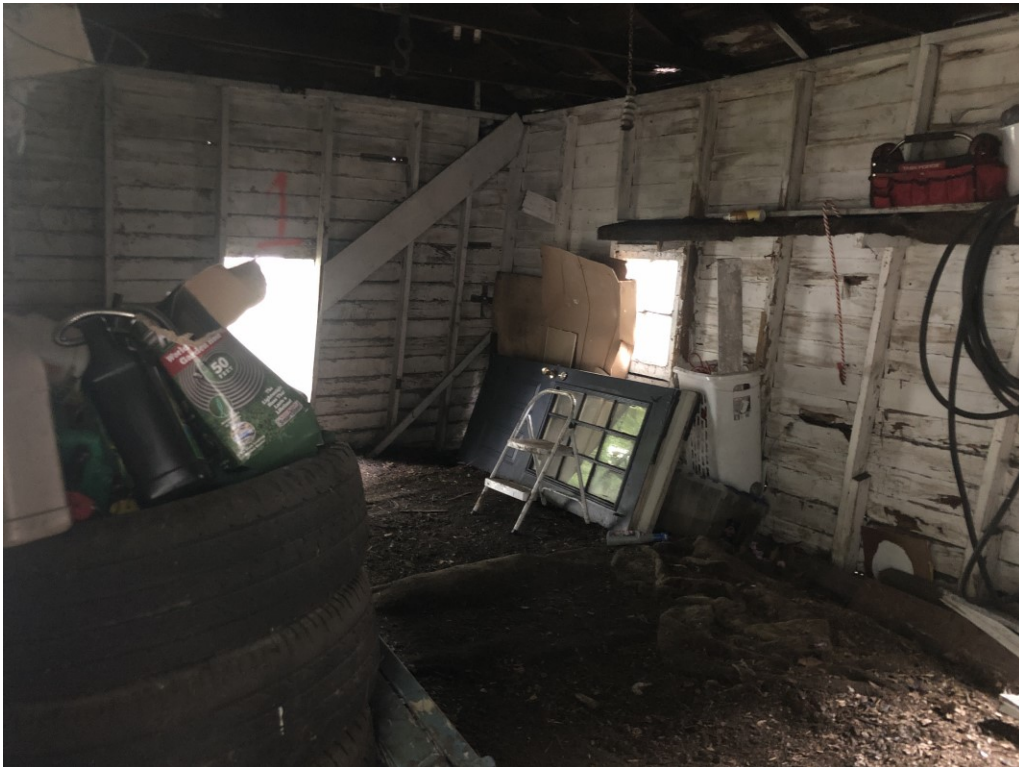
View of the garage interior (FS-1)
