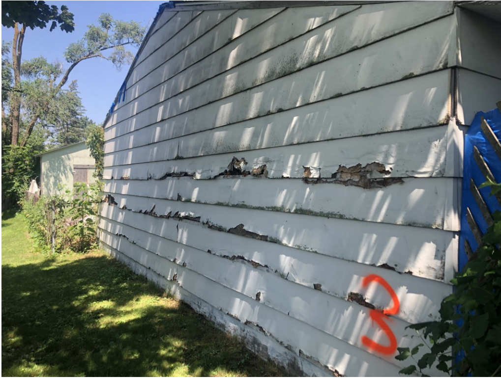
View of the west side of the garage exterior (EA-3)
