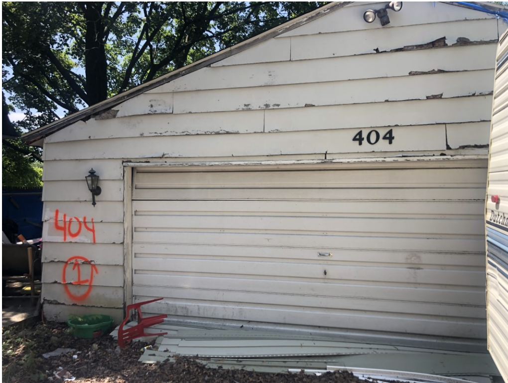
View of the east side of the garage exterior (EA-1)
