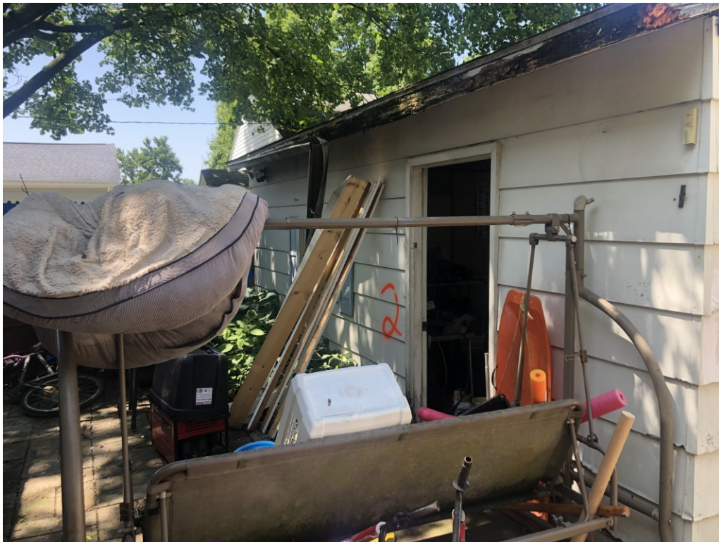
View of the south side of the garage exterior (EA-2)
