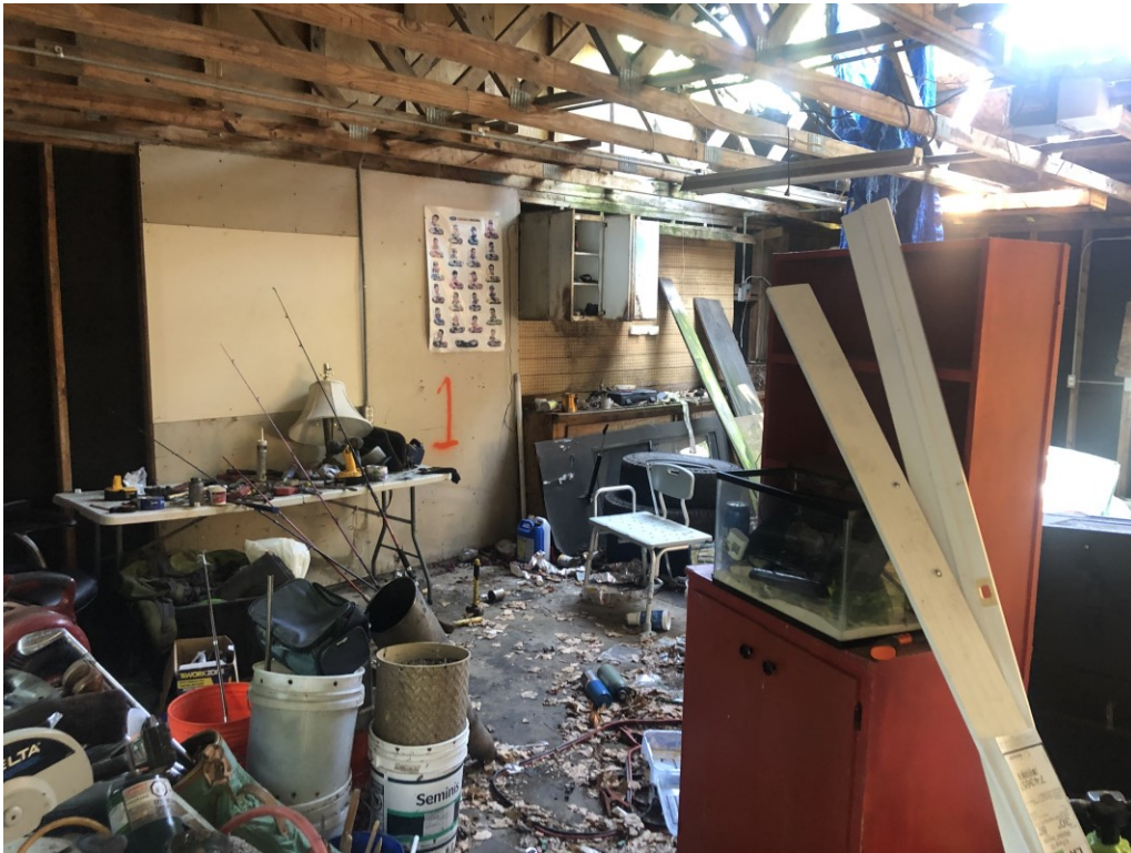
View of the garage interior (FS-1)
