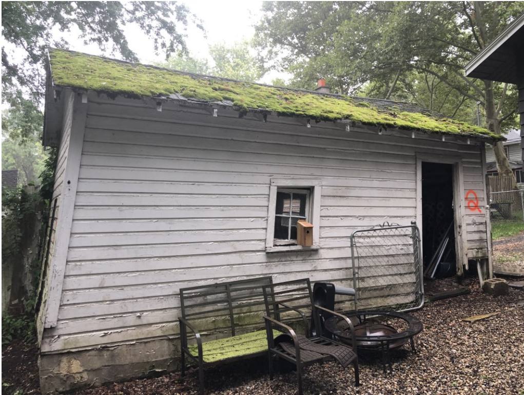
View of the north side of the garage exterior (EA-2)
