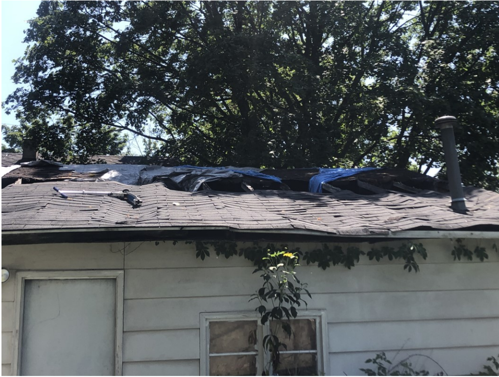
View of the garage roof (EA-5)
