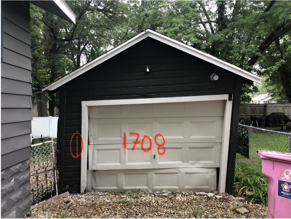
View of the west side of the garage exterior (EA-1)
