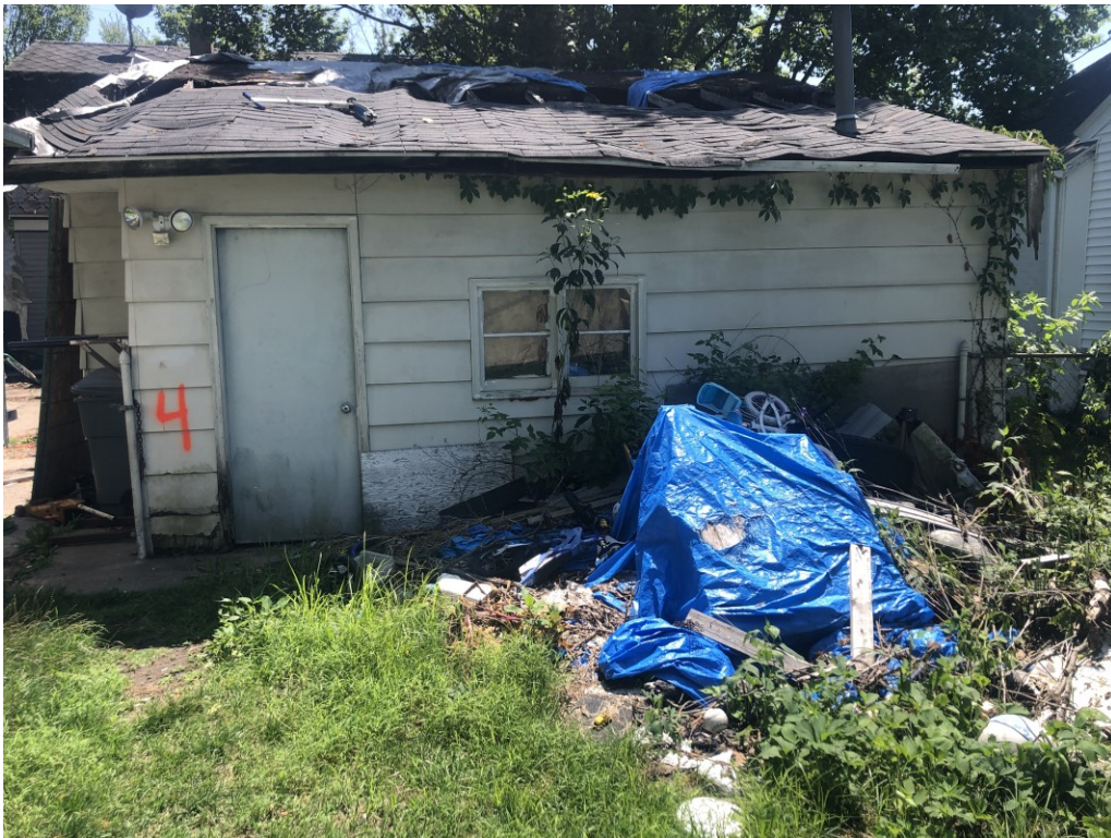
View of the north side of the garage exterior (EA-4)
