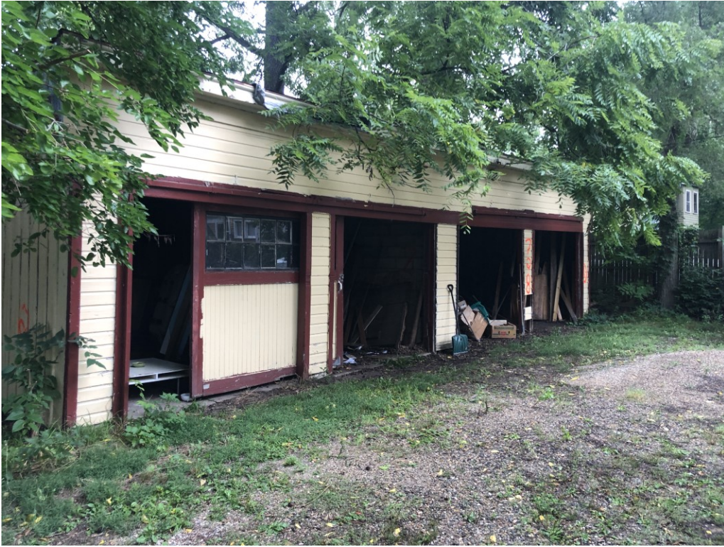
View of the south side of the garage exterior (EA-1)
