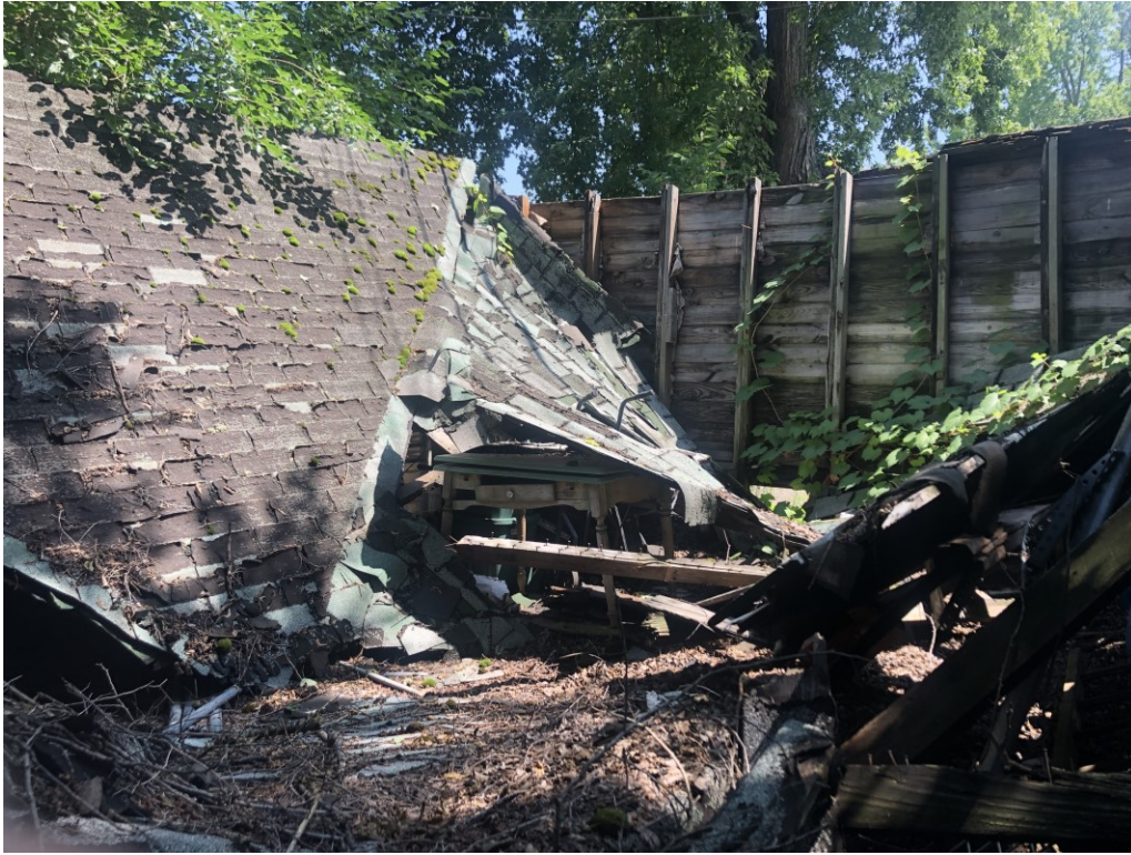
View of the garage interior (FS-1)
