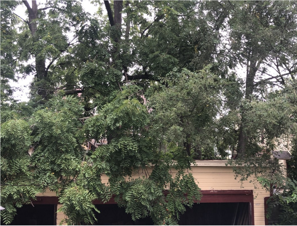
View of the garage roof (EA-5)
