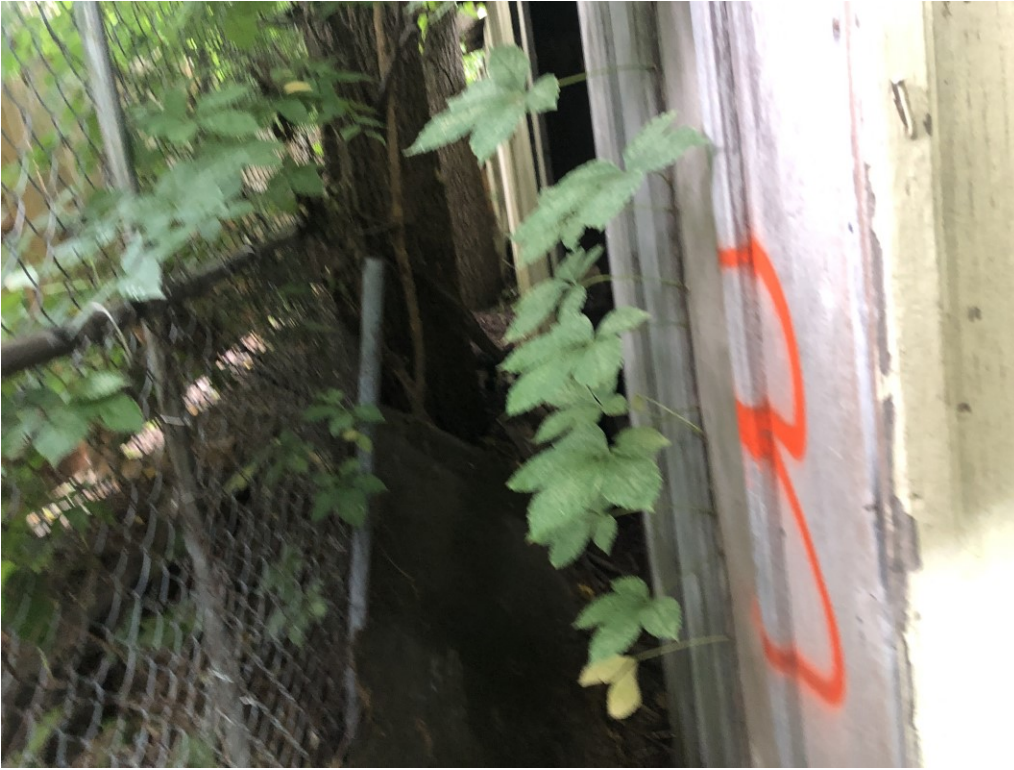
View of the north side of the garage exterior (EA-3)
