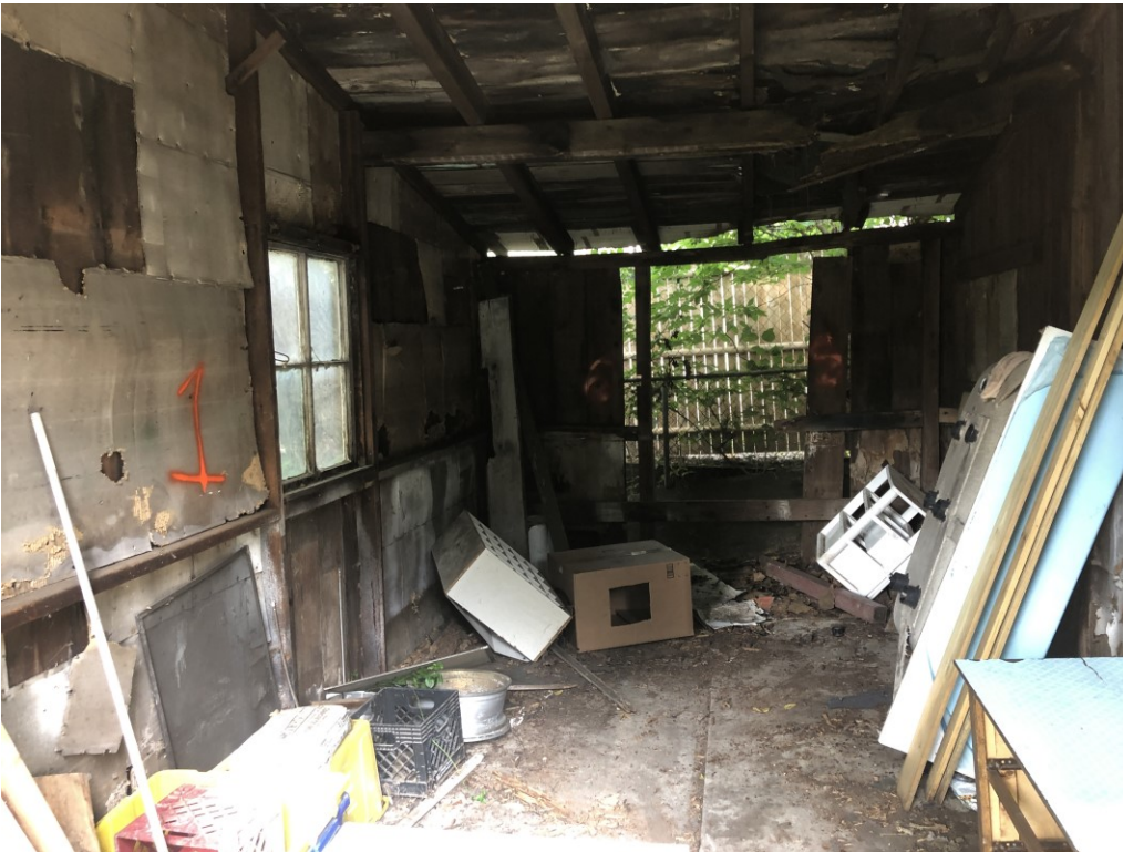
View of the garage interior; bay 1 (FS-1)
