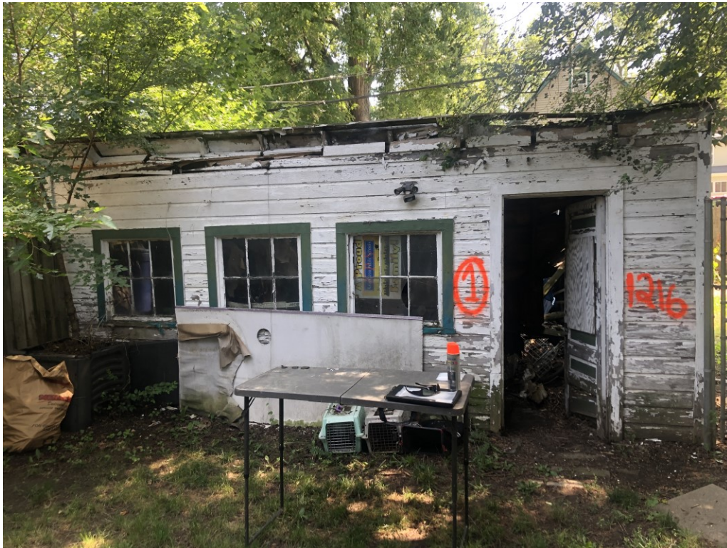
View of the north side of the garage exterior (EA-1)
