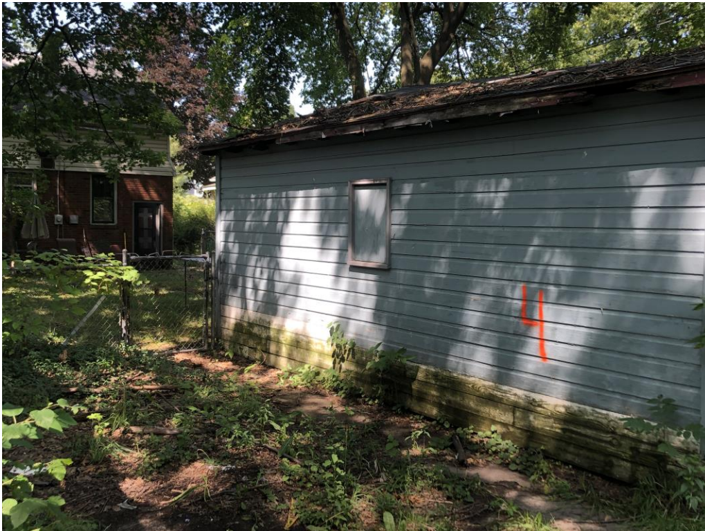
View of the west side of the garage exterior (EA-4)
