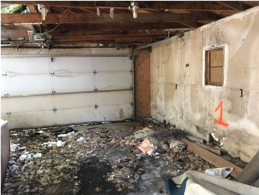
View of the garage interior (FS-1)
