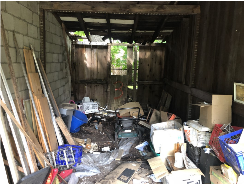
View of the garage interior; bay 3 (FS-3)
