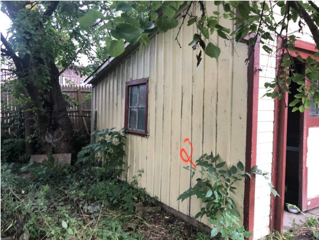
View of the west side of the garage exterior (EA-2)
