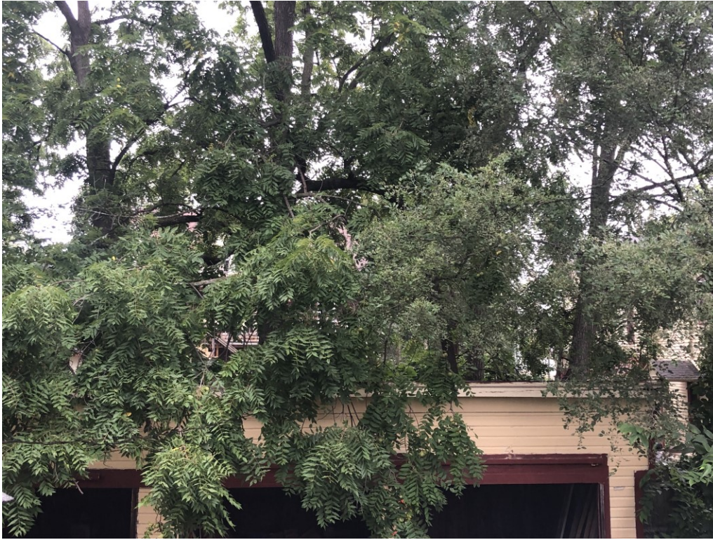
View of the garage roof (EA-5)
