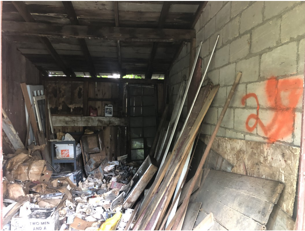
View of the garage interior; bay 2 (FS-2)
