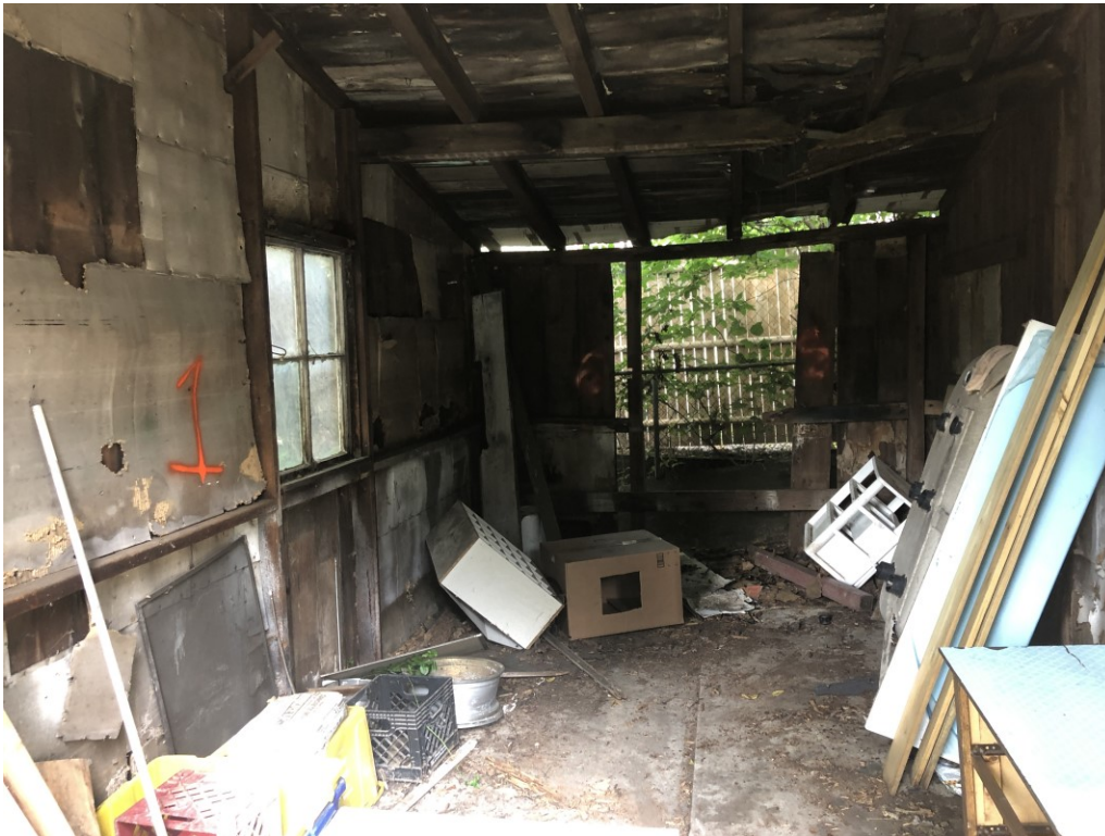
View of the garage interior; bay 1 (FS-1)
