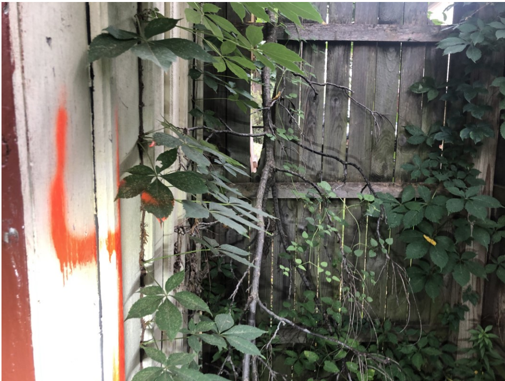
View of the east side of the garage exterior (EA-4)
