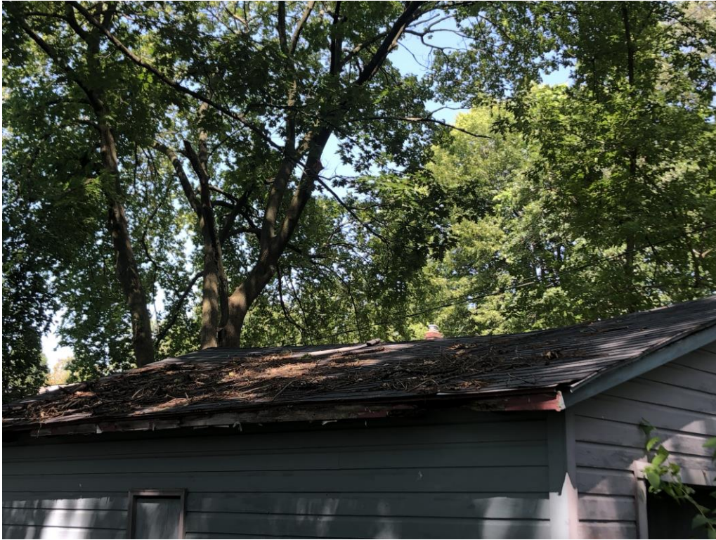
View of the garage roof (EA-5)
