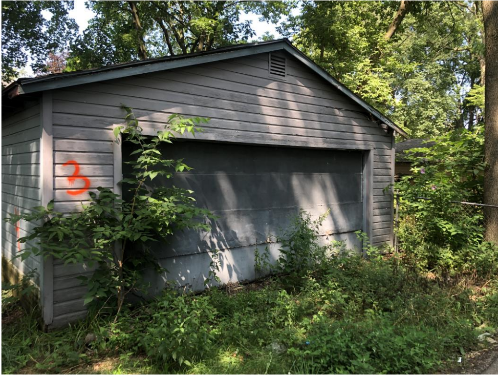
View of the south side of the garage exterior (EA-3)
