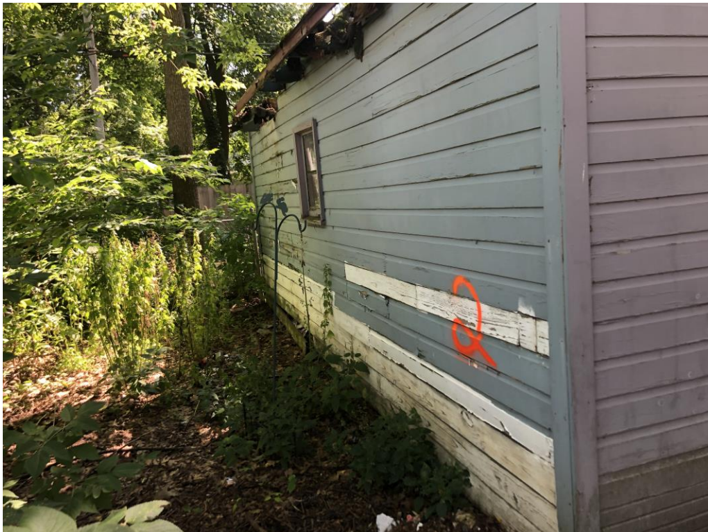
View of the east side of the garage exterior (EA-2)
