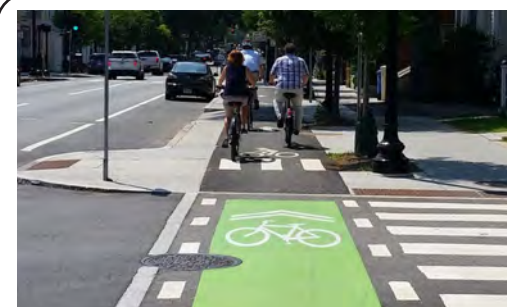
ASPHALT RAISED BIKE LANE ALTERNATIVE 1 ONLY
