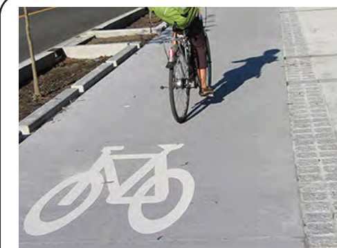
CONCRETE RAISED BIKE LANE
