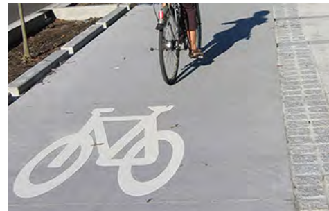
CONCRETE RAISED BIKE LANE
