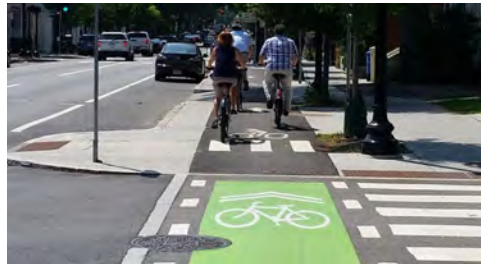
ASPHALT RAISED BIKE LANE
