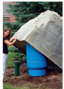
Place Mock Rock Over 8" DIP and 2" HDPE to Conceal Autoflusher Discharge https://allmockrocks.com/ *Minimize Mock Rock Size to Maximum Extent*
