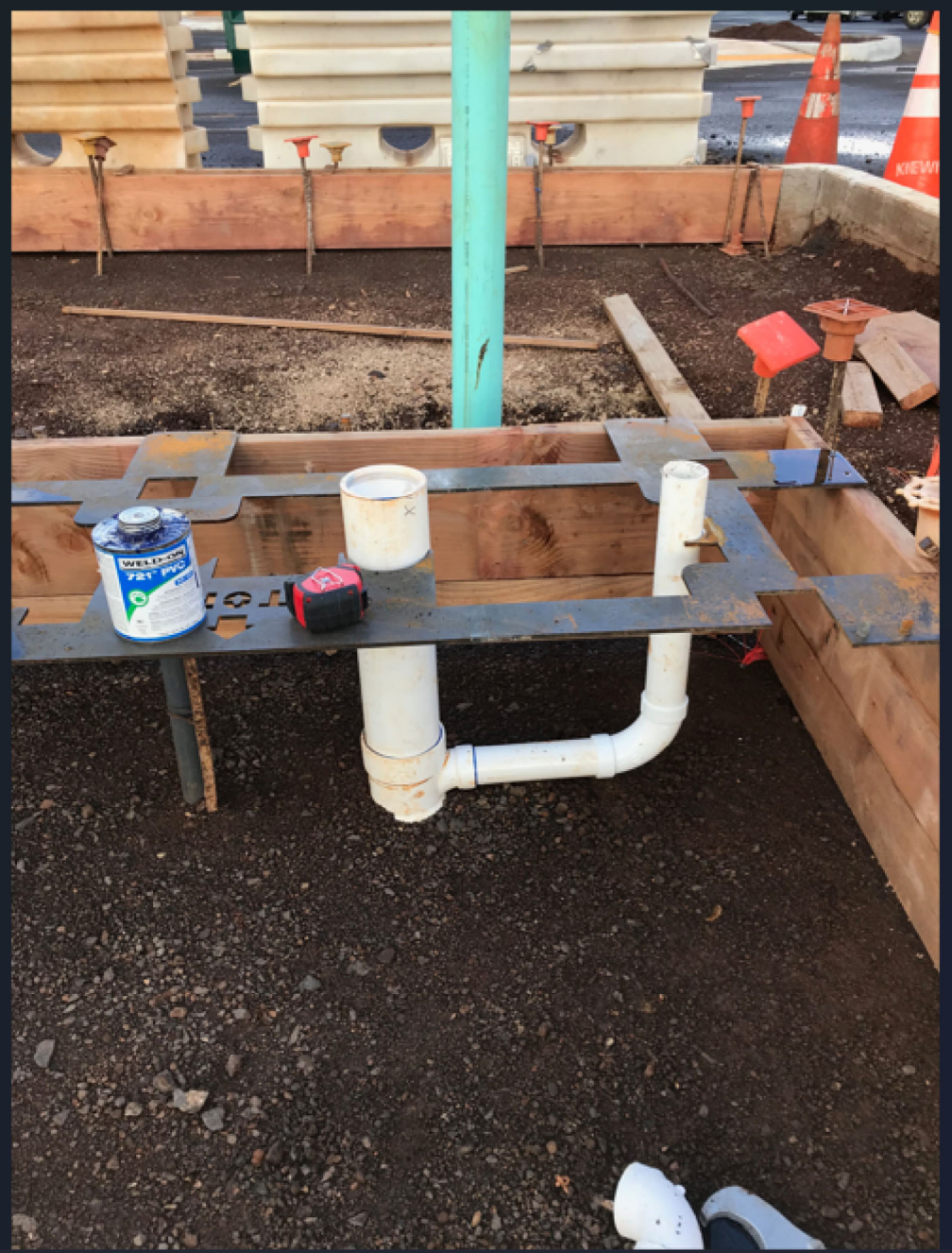
Jig Detail - Recessed Handwash Drain
