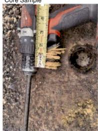
Concrete deck (sloped west to east), 3/4" fiberglass smooth BUR, 3/4" fiberglass, 4 ply BUR with gravel.
