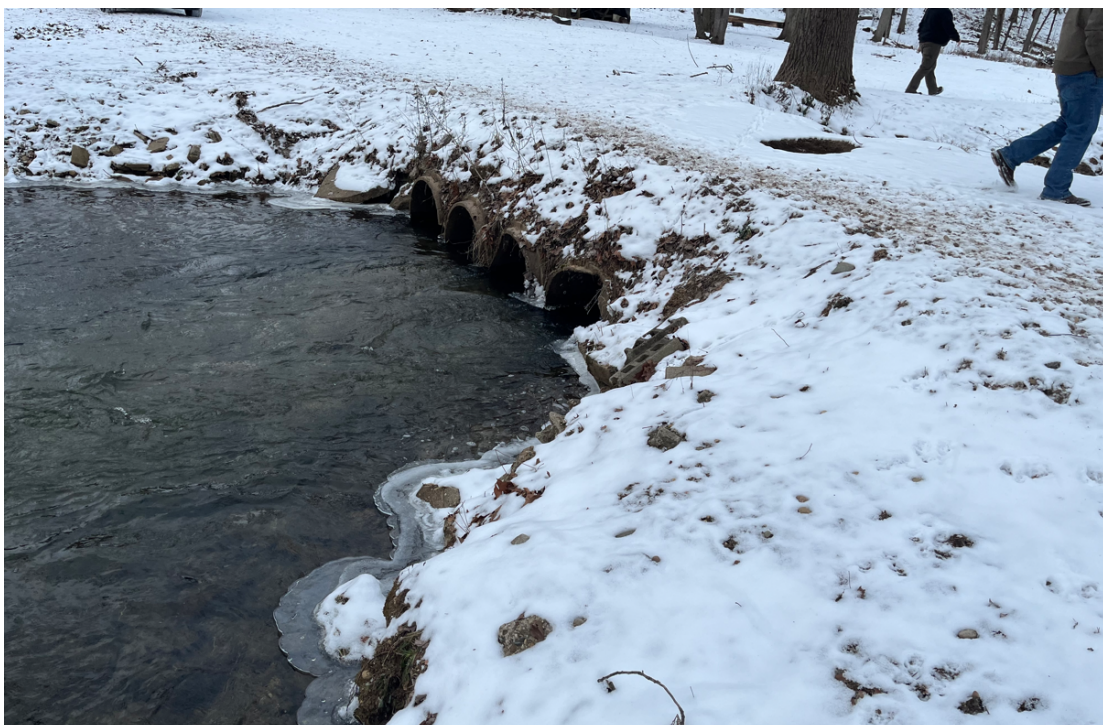
Current Condition, west side
