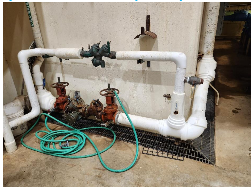
Photo 3 – Existing Piping with Ball Valve
