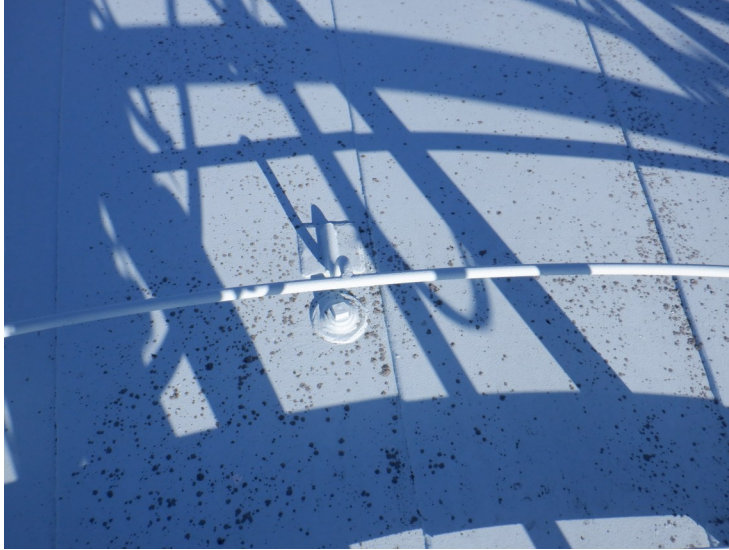
22) The roof painter's railing and rigging couplings are in good condition.
