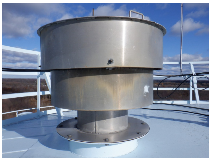
15) The pressure vacuum vent is in good condition.
