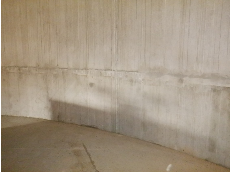
31) Typical column section with no deterioration.
