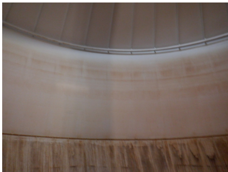
51) The sidewall coating is in good condition with no significant deterioration.
