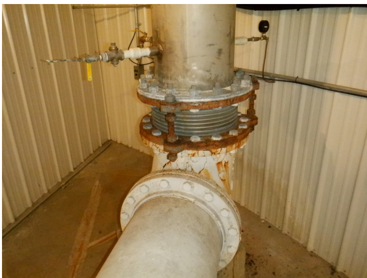
30) The bellows expansion joint is in good condition.
