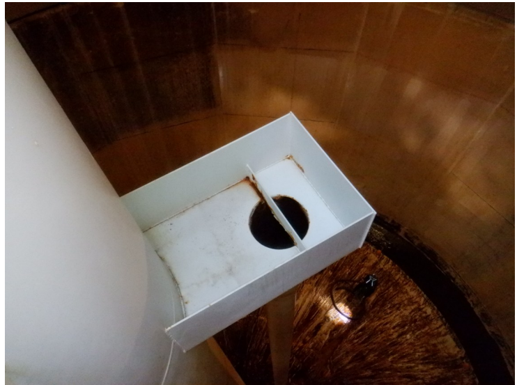
53) The overflow weir box is in good condition.
