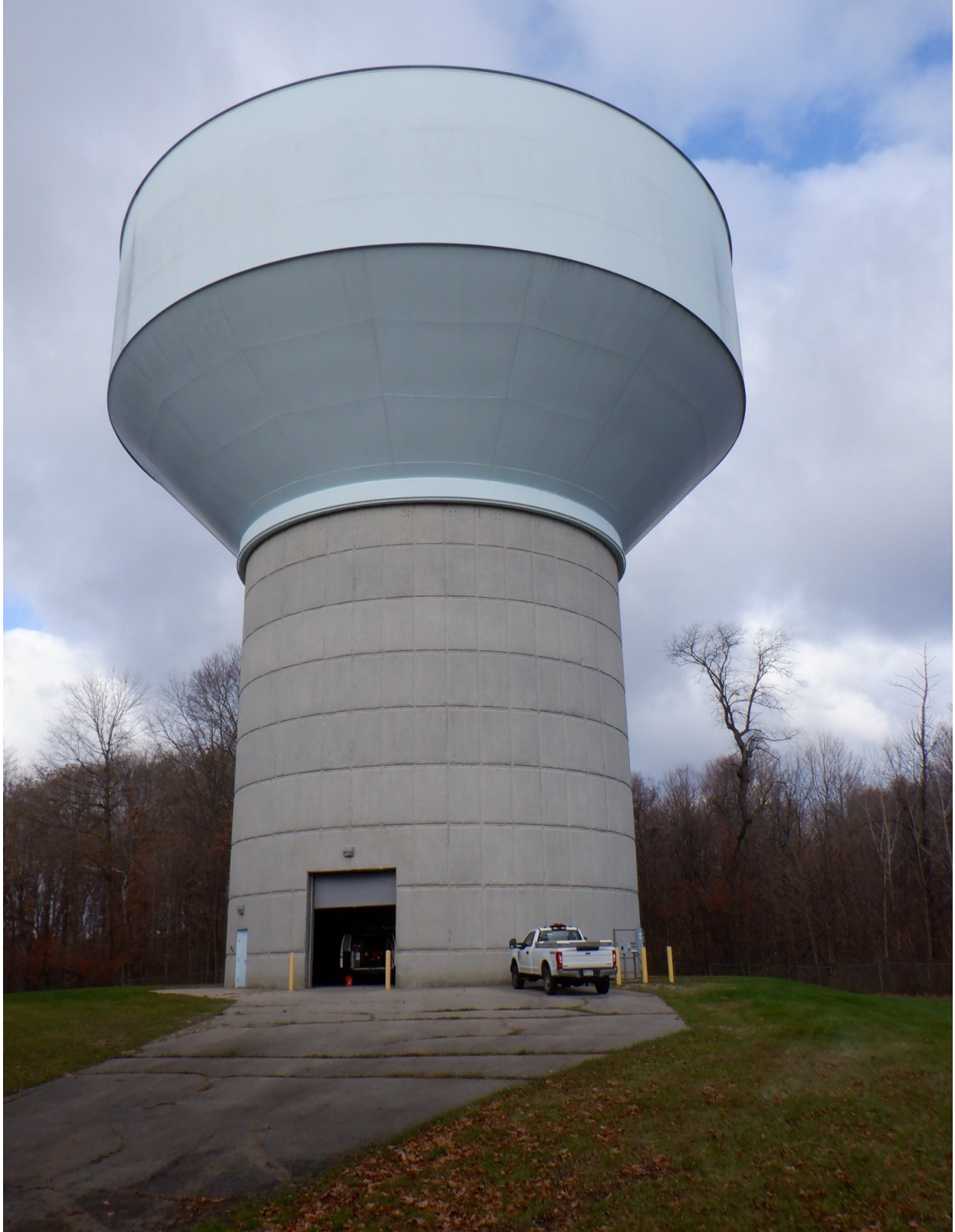
2,500,000 gallon composite (Beech Avenue) located in Kalamazoo, Michigan.
