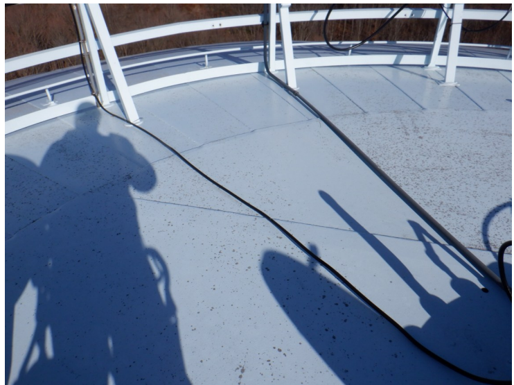
26) Roof coating inside the handrail is in good condition.
