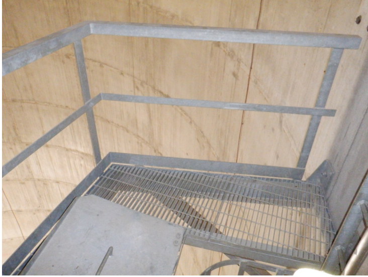
34) Typical step-off platform is in good condition.
