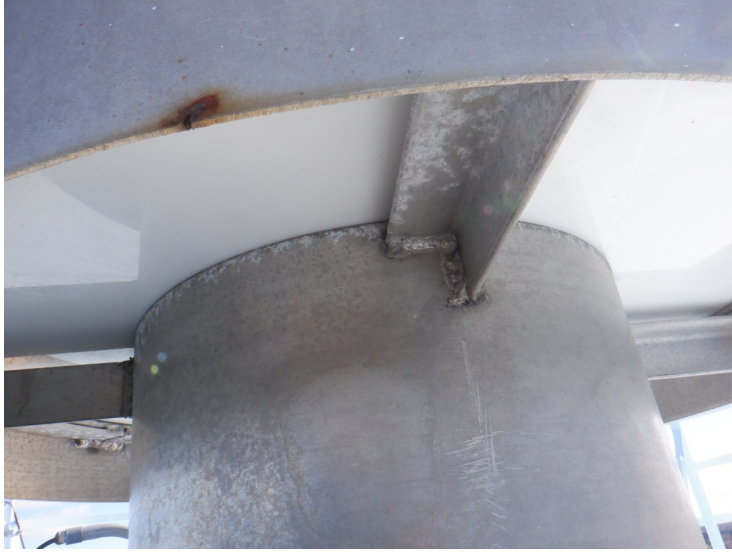
16) The pressure plate is in good condition. The plate was found to be properly aligned during the inspection.
