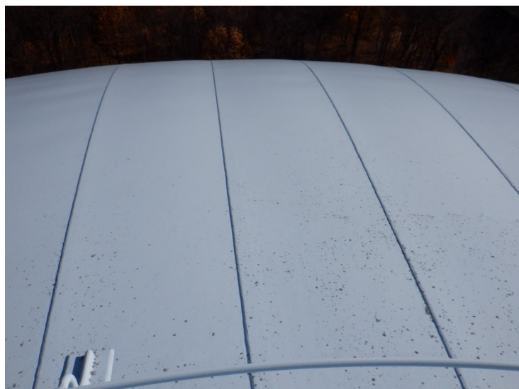
24) The roof coating is in good condition overall.
