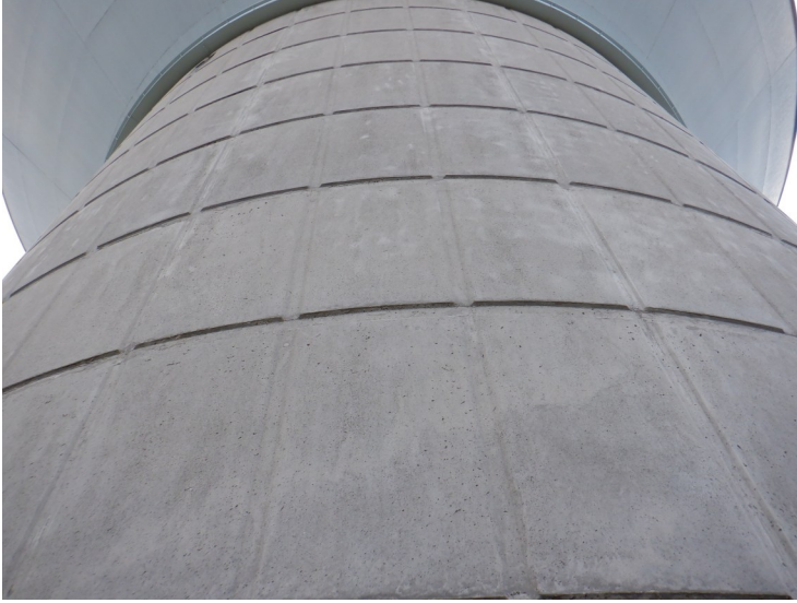
7) Typical column section with no significant deterioration.
