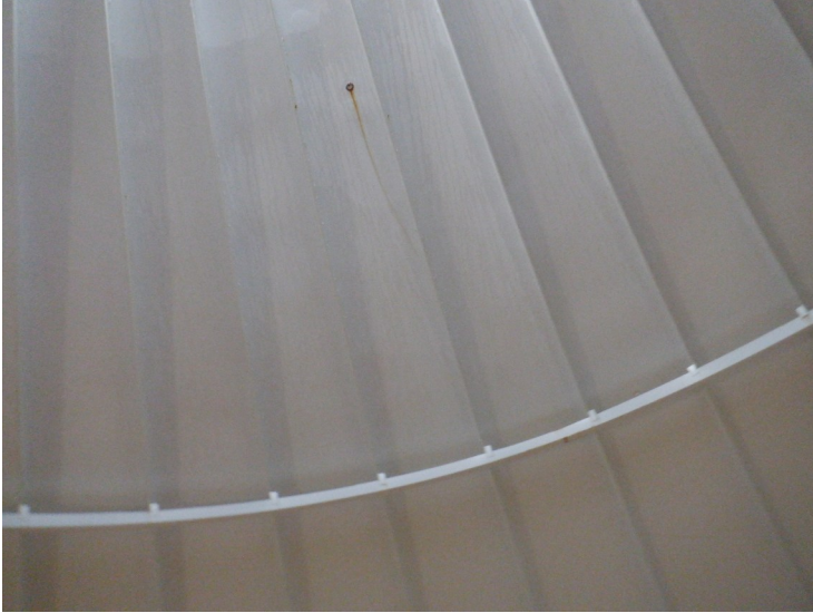
49) The roof coating is in good condition overall.
