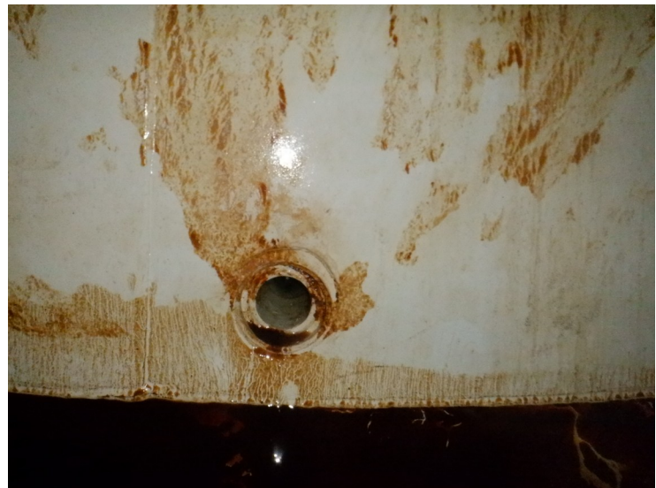
65) The mud valve drain appears to be in good condition.
