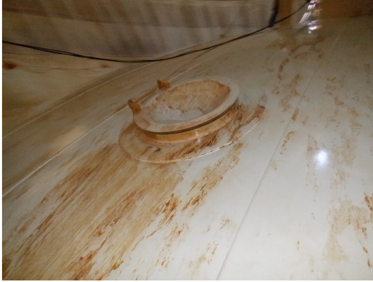
64) The wet interior manway cover is in good condition.
