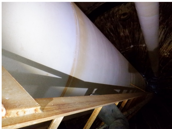
54) The access tube coating is in good condition overall.
