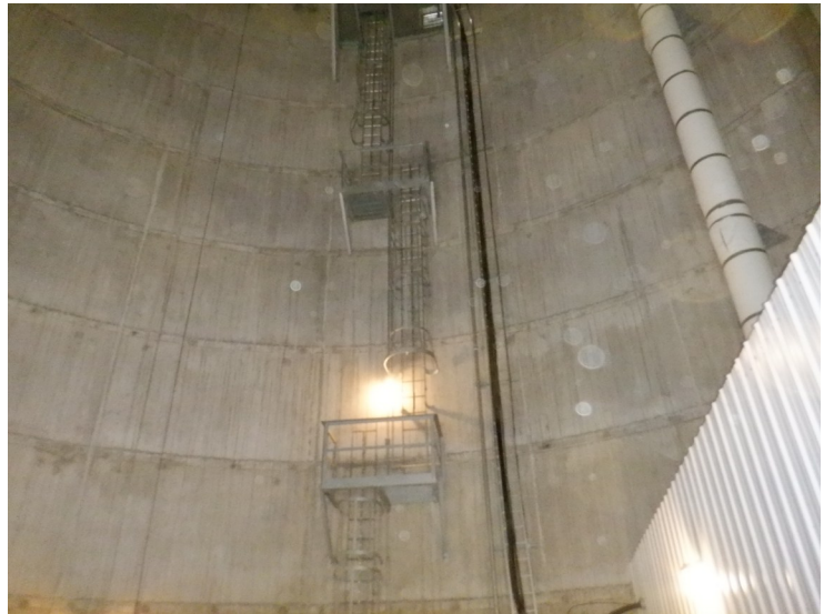
32) The column ladders and step-off platforms are in good condition.
