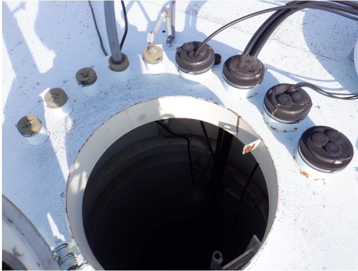
13) The dry interior roof hatch is in good condition.
