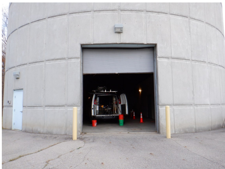
6) The retractable overhead door is in good condition.
