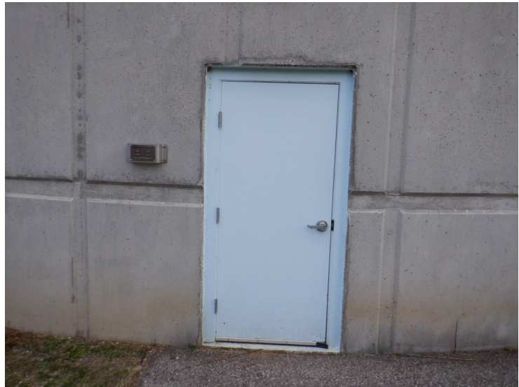
5) The column service door is in good condition.
