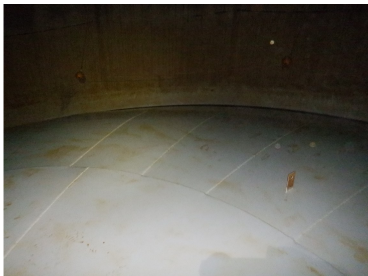
60) The domed bottom coating is in good condition overall.
