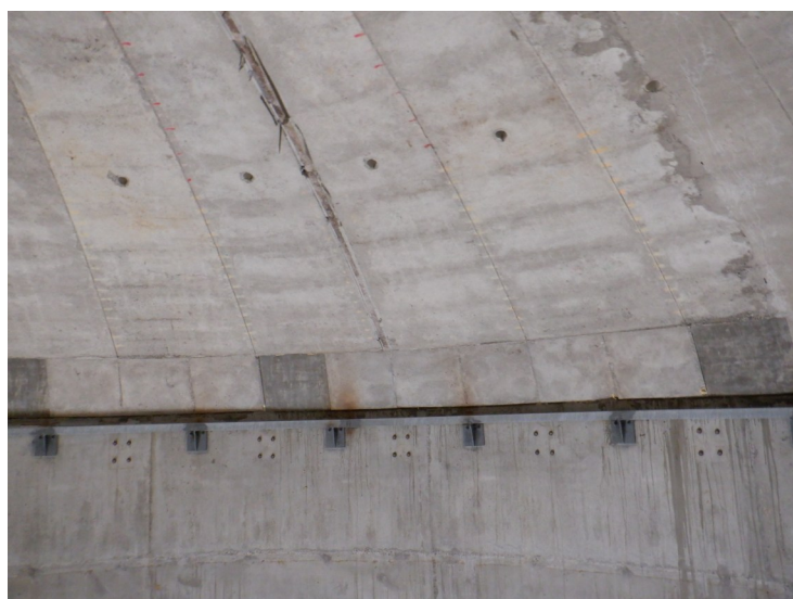
39) The concrete dome is in good condition with no significant deterioration.
