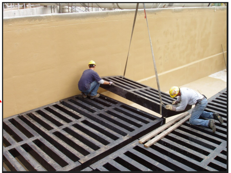
Support Grading Installation
