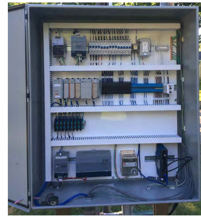
SAMPLE METERING PANEL LAYOUT
