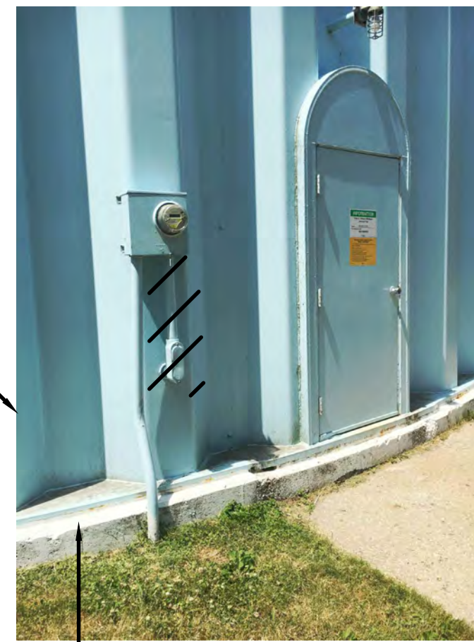
CORE HOLE(S) AS REQUIRED FOR NEW CONDUITS. SEE NOTE NO. 10, AND NOTE NO. 12 BELOW.
