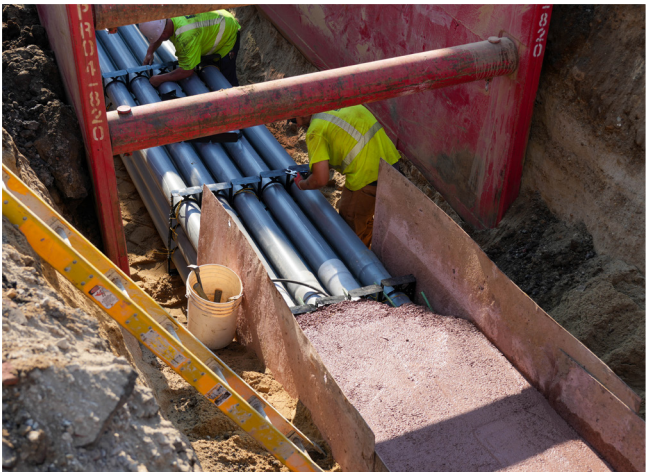
Left: New water main on Kalamazoo Ave is connected to the water system. The old main being replaced is visible where it has been cut. Top: Crews install an electrical duct bank on Kalamazoo Ave. Fifteen conduits encased in concrete will eventually allow overhead power lines to move underground.
