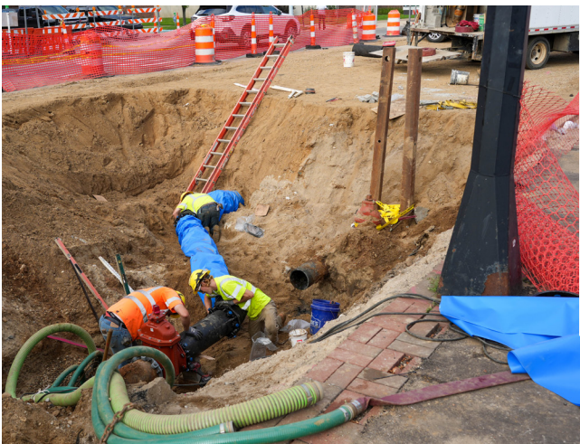
Left: New water main on Kalamazoo Ave is connected to the water system. The old main being replaced is visible where it has been cut. Top: Crews install an electrical duct bank on Kalamazoo Ave. Fifteen conduits encased in concrete will eventually allow overhead power lines to move underground.
