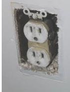
Electrical receptacles and switches are not meant to be painted. Over time plugging things in and out can transfer paint chips into the receptacle and cause a fire or malfunction. If inspectors see painted switches and receptacles, replacement will be necessary.
